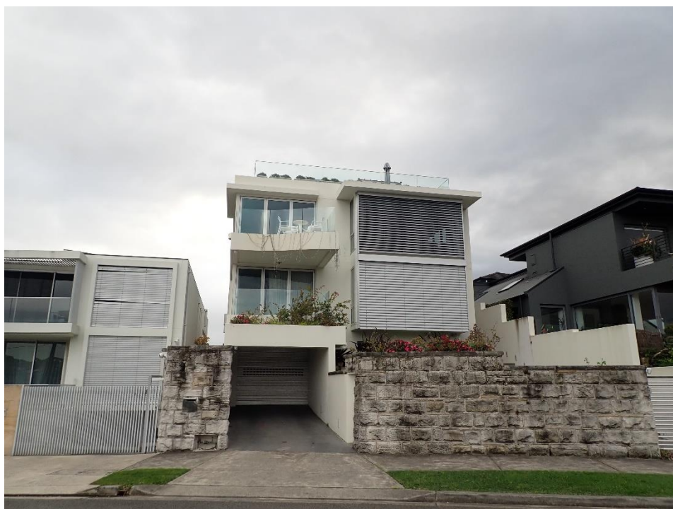
Figure 10 – Photo opposite 10 Larkin Street – existing awning structure not visible
