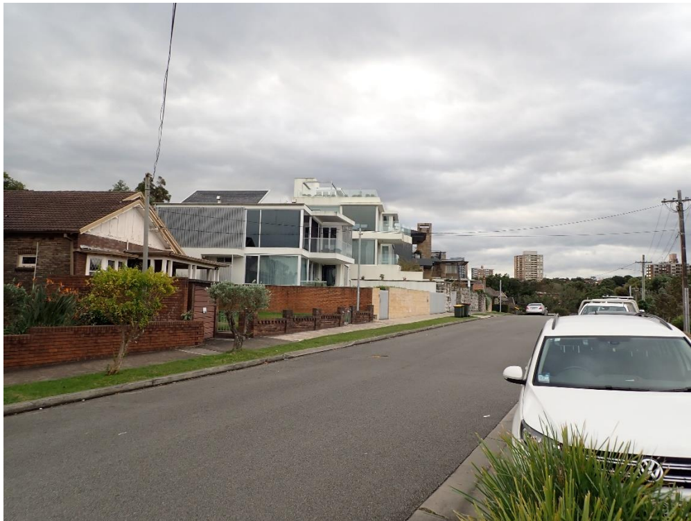
Figure 12 – Photo opposite 4 Larkin Street – awning structure increasingly visible
