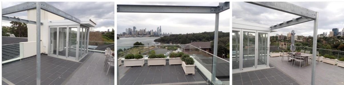
Figures 6, 7 & 8 – Photo of rooftop subject to the retractable awning
