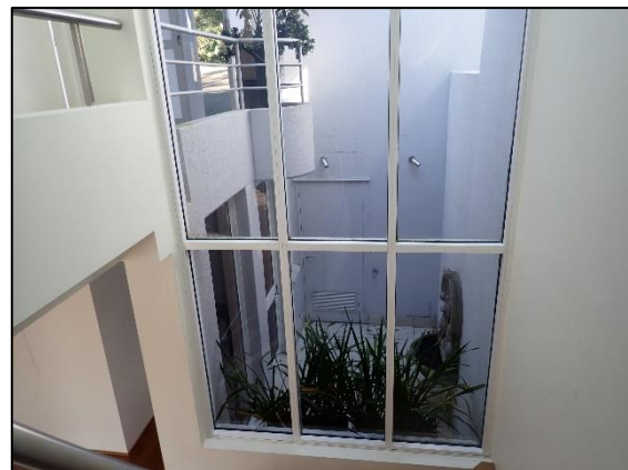
Figure 6. View of the central light well, the location of the proposed lift.
