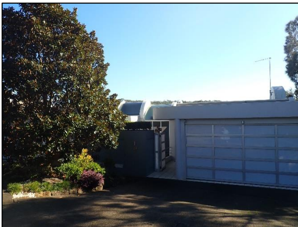
Figure 5. View of the site from Folly Point road.
