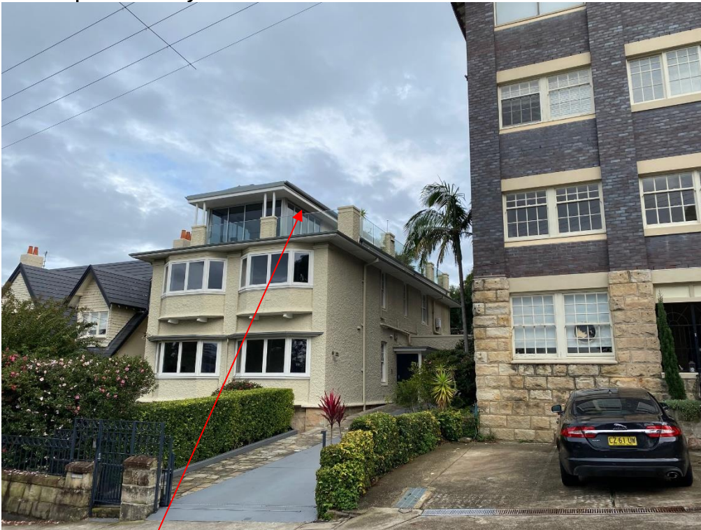
Rooftop terrace and open pavilion – 16 Cremorne Road
