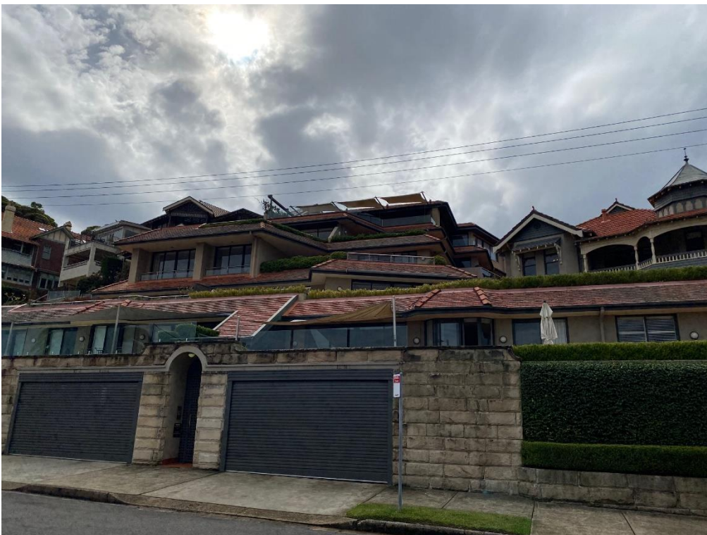
Open terraces and balconies – 25 Milson Road
