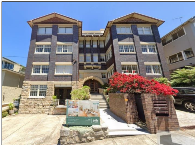
Figure 5. View of the site from Cremorne Road.
