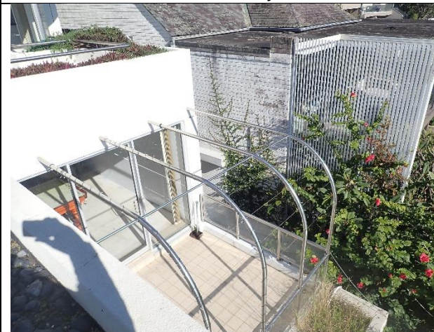
Figure 6. View looking west over the Level 2 north-west corner balcony.
