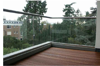
BL1 SEMI- FRAMELESS, CLEAR GLASS BALUSTRADE WITH ROUND S/S TOP RAIL
