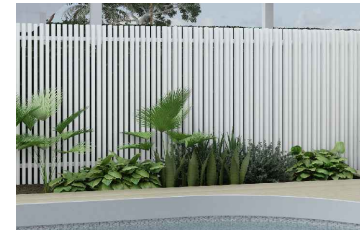
MT1 WHITE POWDERCOATED VERTICAL METAL LATTICE FINISH
