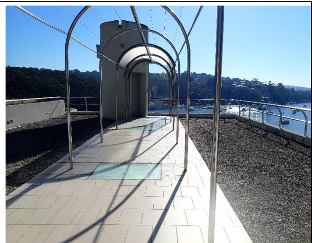
Figure 5. View looking north across the roof level and access (Level 5).
