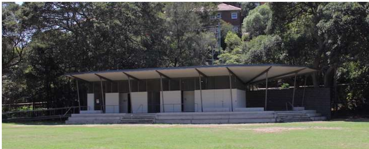
Site Photo: Existing amenities building
