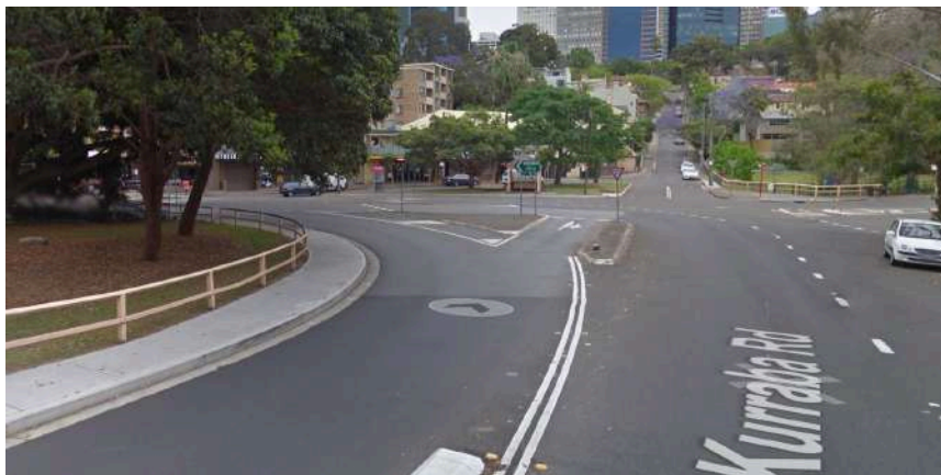
Site Photo: Area of the proposed integrated traffic and public domain project viewed west from Kurraba Road
