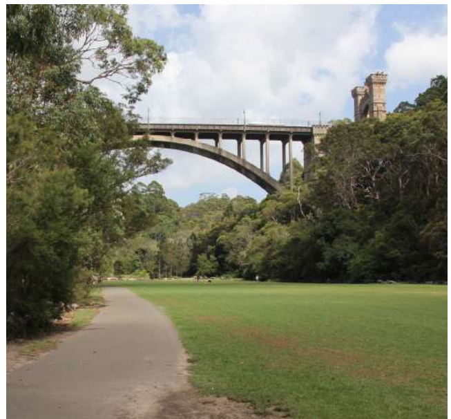
Site Photo: Suspension Bridge
