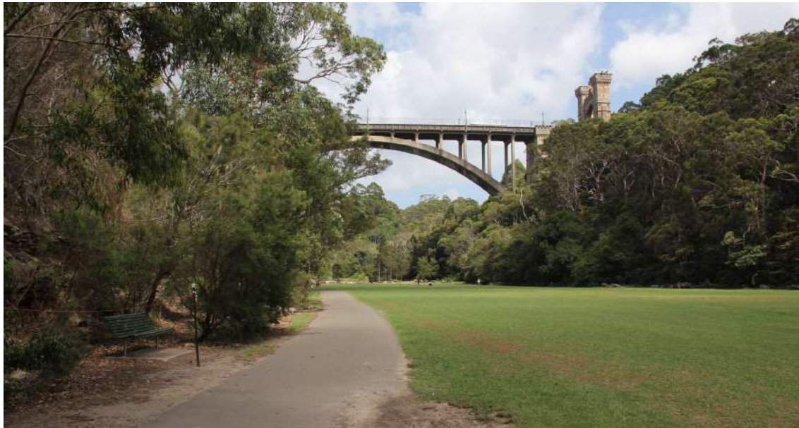
Site Photo: View from Brothers Avenue to open space / playing field No. 1
