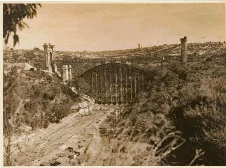
Historic Photo: Construction of Arch bridge to replace suspension bridge 1938 copyright State Library of NSW
