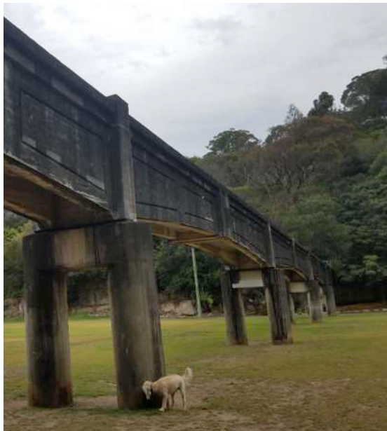
Site Photo: Sewer Aqueduct
