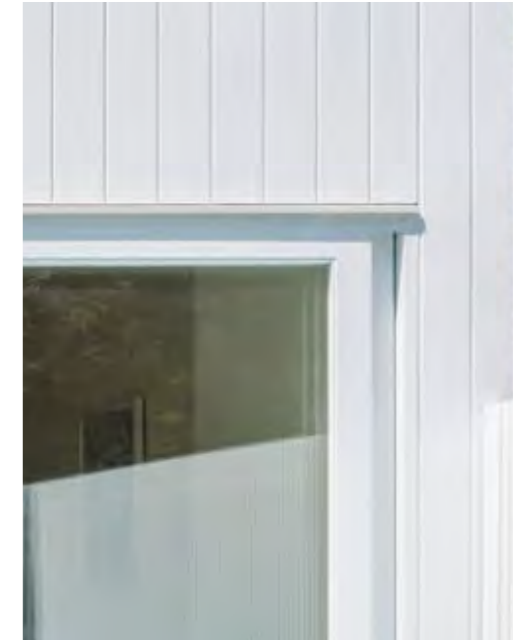
WB. 'Natural White' vertical weatherboard cladding TW. 'Vivid White' timber frame windows and doors Source: The Local Project
