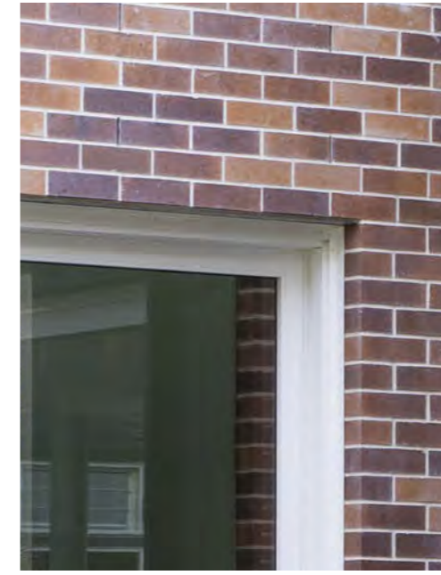
BW. Bricks to match existing TW. 'Vivid White' timber frame windows and doors Source: Cedar and Suede
