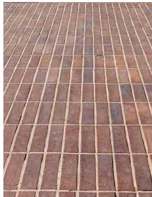
BP. Brick paving to patio to match existing bricks Source: Manna Gum Building and Garden Supplies
