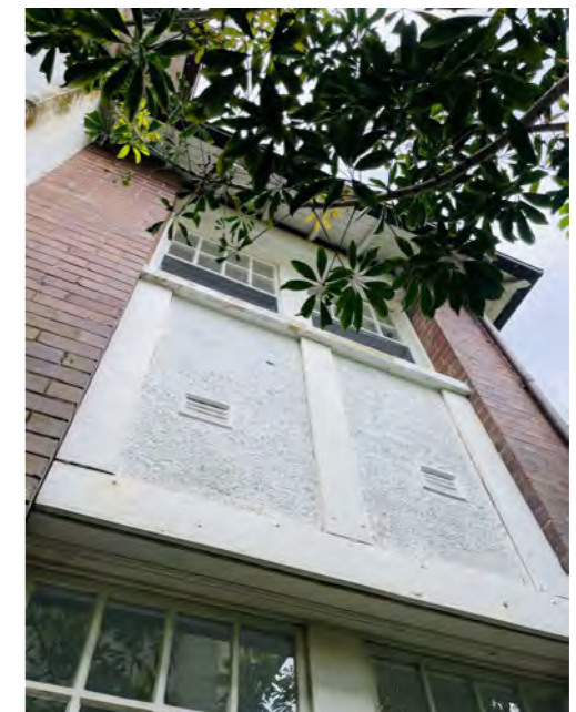
12. Restore timber panelling 2. Retain and restore white stucco
