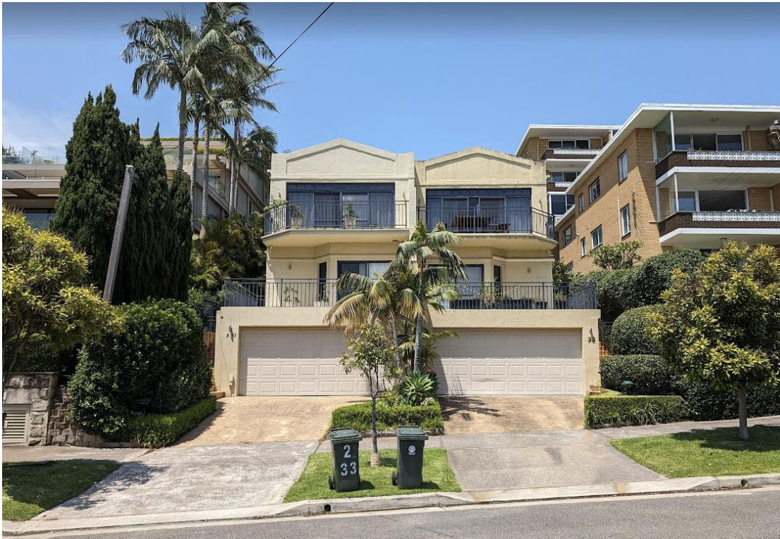
Medium density development on the southern side of Grasmere Road.
