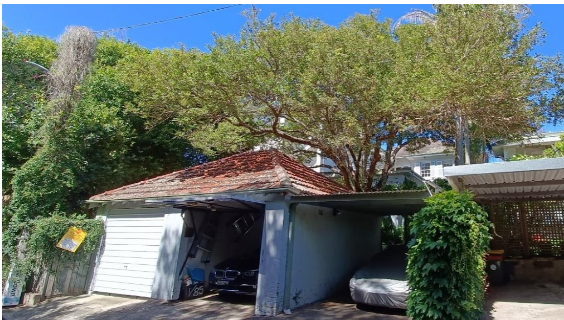
Figure 9: Subject site – As seen from Kareela Lane showing the existing two car garage and the single carport
