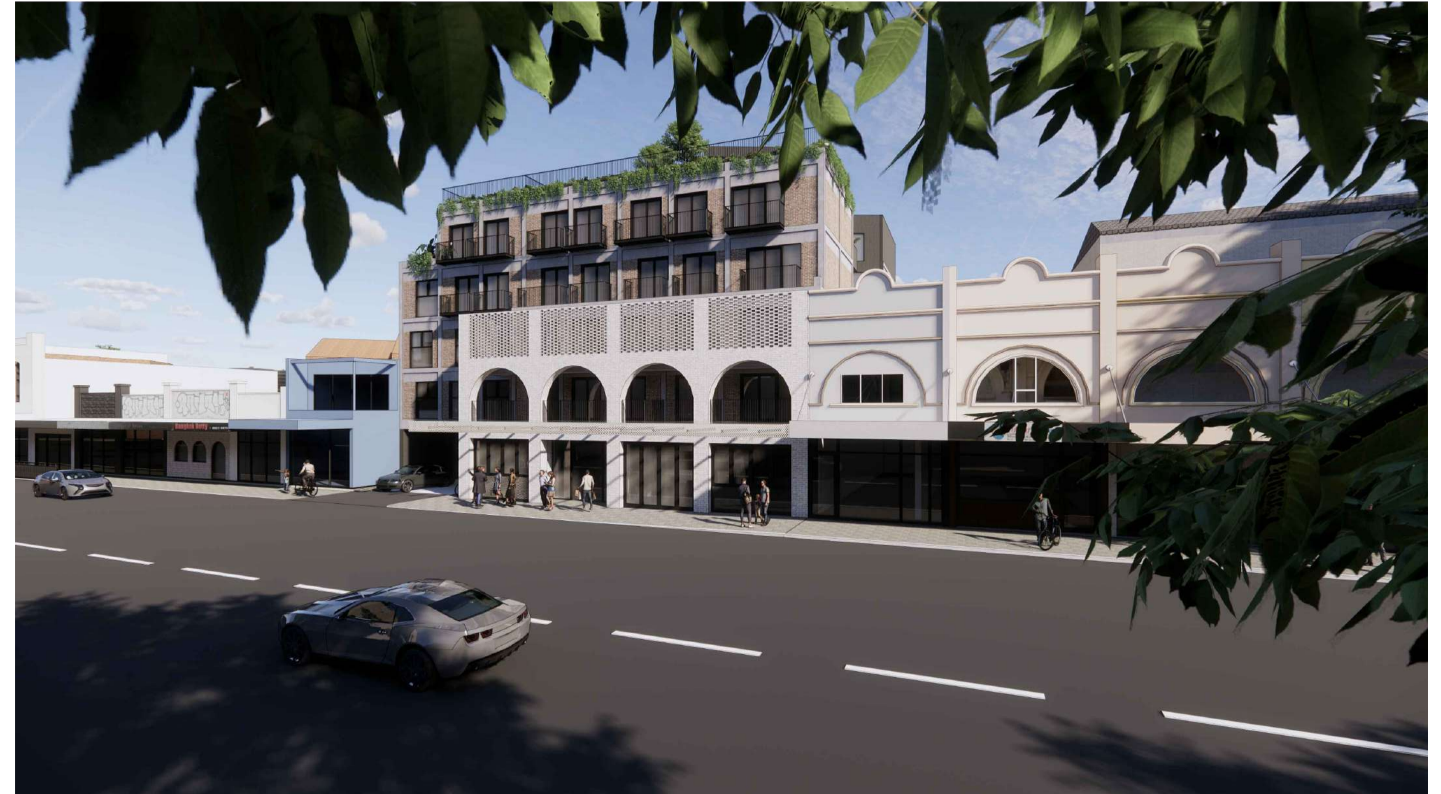
VIEW FROM MILITARY ROAD TO NORTH-EAST
