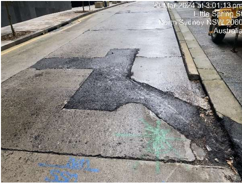
Photos – typical images of failed road sections to be reconstructed
