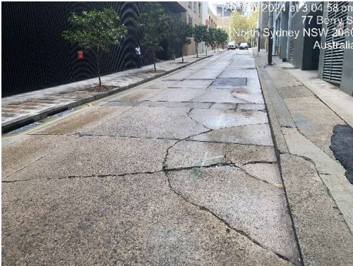
Photos – typical images of failed road sections to be reconstructed
