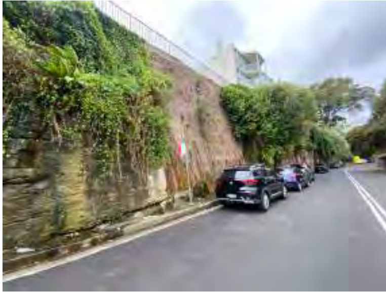
Figure 21: Southern boundary of No.3 Warung Street. Note the brickwork retaining wall above the 1909 sandstone cutting.
