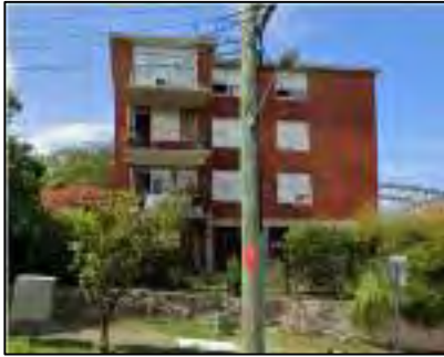
Figure 11: Existing western façade
