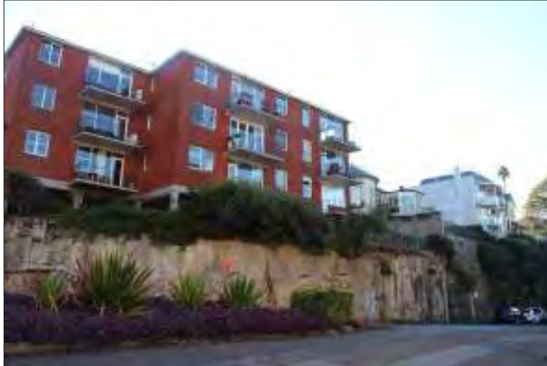
Figure 3: The Henry Lawson Drive boundary. The curve was cut to accommodate a steady gradient for the tramline.
