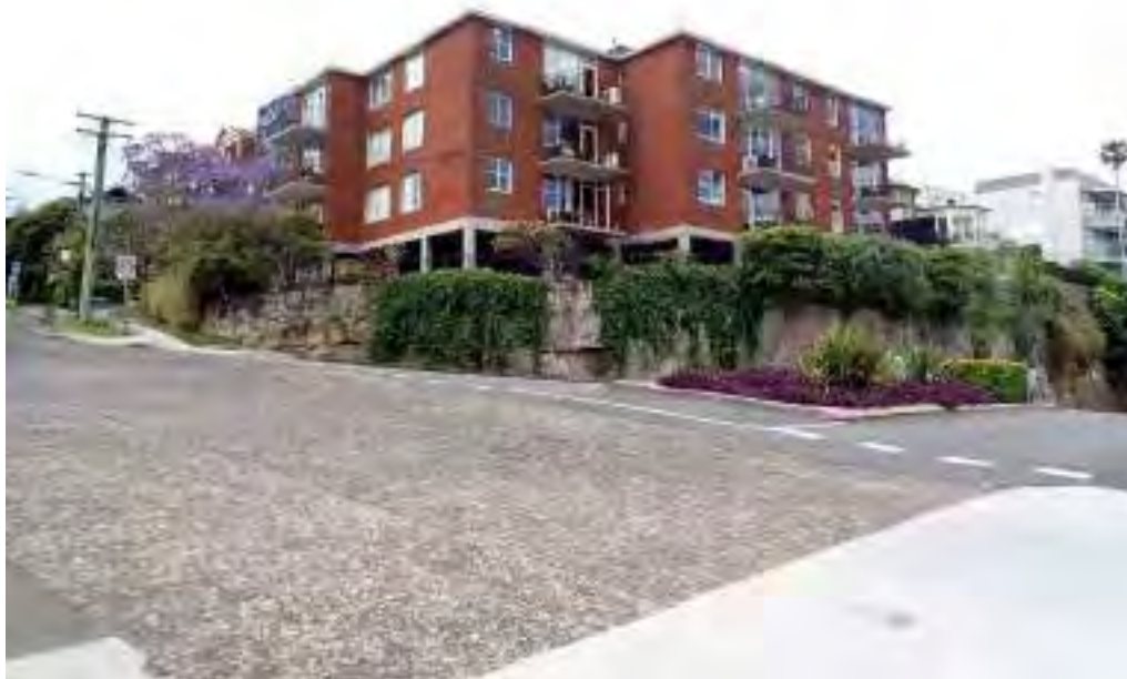
Figure 5 – Photo of the existing RFB as viewed from Blues Point Road
