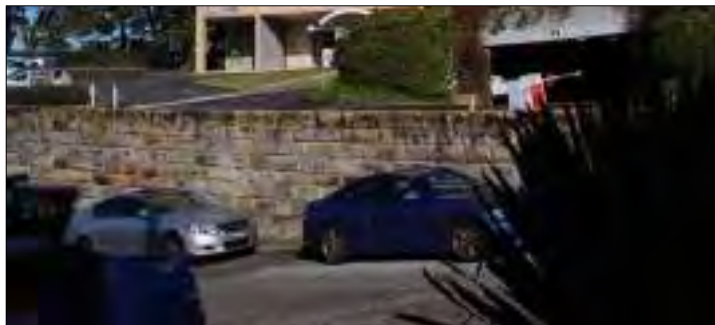
Figure 41: Stone retaining wall.
