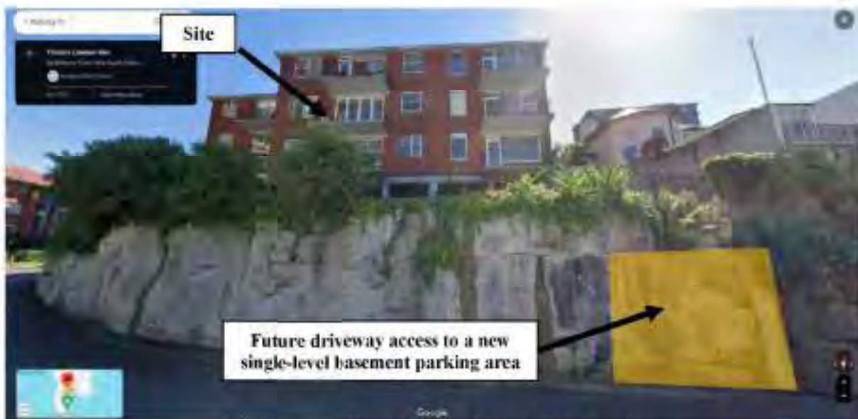
Site view from Henry Lawson Avenue, facing north
