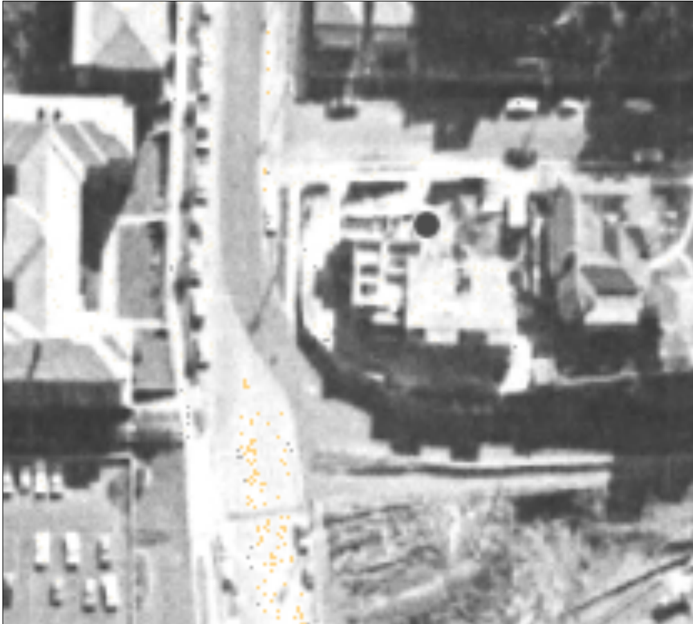
Figure 30: 1965 aerial showing the site under construction.
