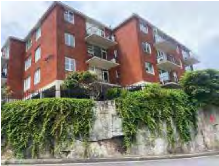
Figure 20: The northern side of Henry Lawson Avenue showing the road cutting.
