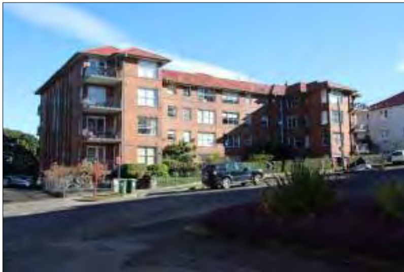
Figure 18: Medium density residential flat building at No. 30-40 Blues Point Road, McMahon's Point.
