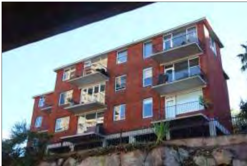
Figure 11: The southern and western elevations.
