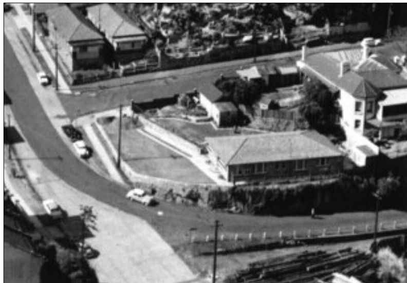
Figure 29: 1958 Aerial view north along Blues Point Road.
