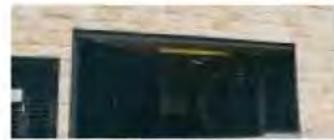
B. BASEMENT GATE. DARK WEATHERED BRONZE FINISH METAL 20 x 20mm SHS @ 40mm CENTRES
