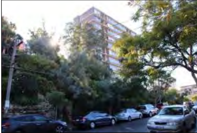
Figure 16: Dwellings directly opposite the subject property.
