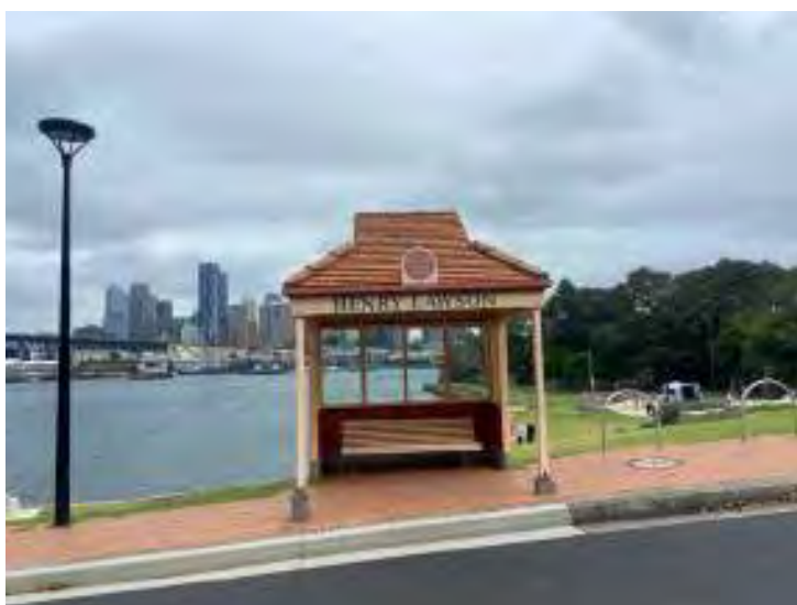
Figure 38: Henry Lawson Bus shelter.
