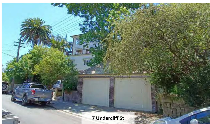
Figure 10: Undercliff Street looking north
