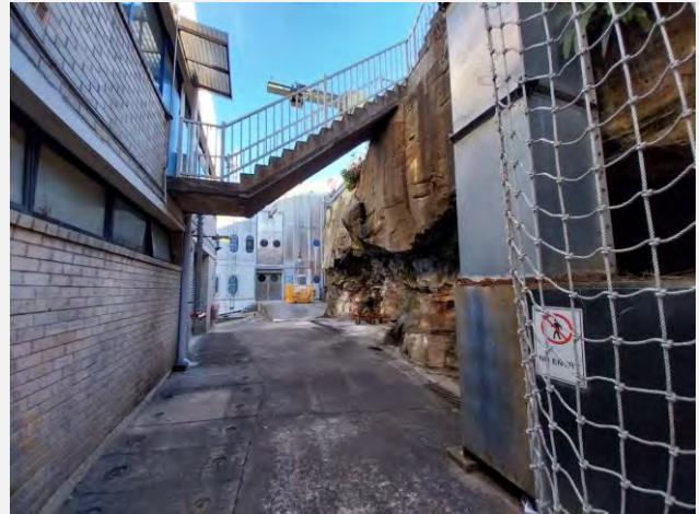
PHOTOGRAPH 2-11 THE CLIFF FACE AND ADJACENT ADMINISTRATION BUILDING ON LEFT (ERM 2023)
