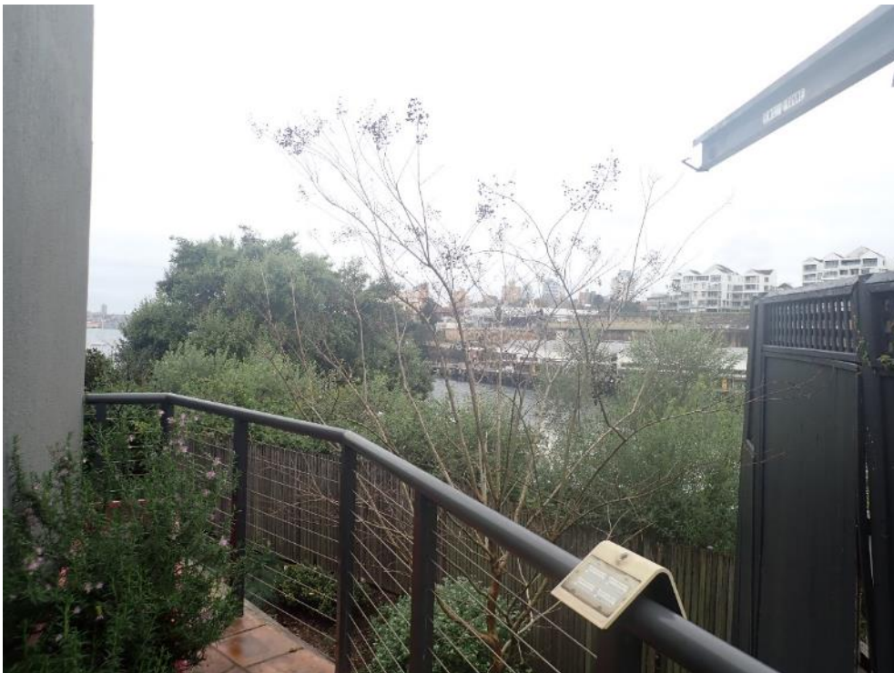
APPENDIX C PHOTO 47 "External Terrace", Unit 6, 2 Hayes Street, Neutral Bay (Photo reference: P8130046)
