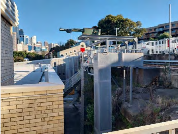
PHOTOGRAPH 2-5 TRAINING STRUCTURE BUILT ON CLIFF WALL (ERM 2023)
