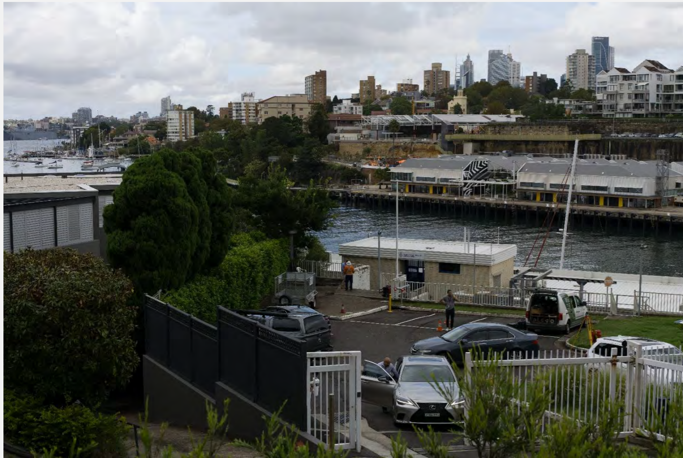
PHOTOGRAPH 6-1 VIEW ONE: MONTEATH AND POWYS IMAGE 0006 – VIEW FROM SOUTHERN END OF NO. 1-5 MANN'S AVENUE LOOKING SOUTH-WEST
