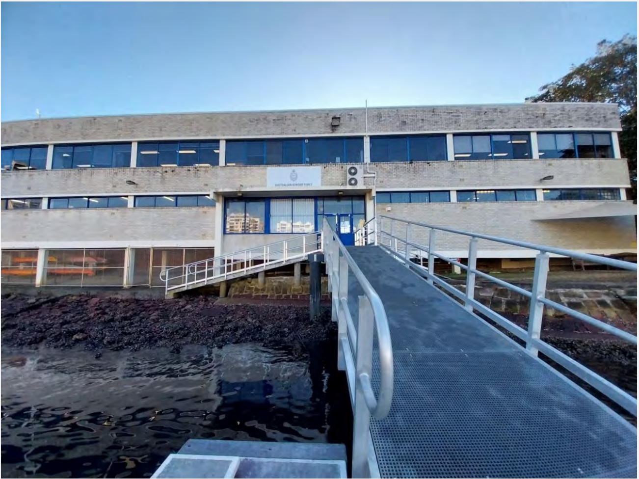
PHOTOGRAPH 2-7 VIEW OF THE ADMINISTRATION BUILDING FROM THE JETTY (ERM 2023)
