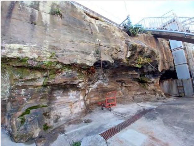
PHOTOGRAPH 2-10 CONCRETE PAVING AT REAR OF ADMINISTRATION BUILDING (ERM 2023)
