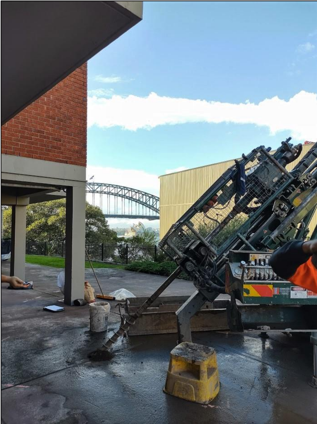
Photograph 1: Track-mounted drilling rig on 45° angled borehole (BH03)
