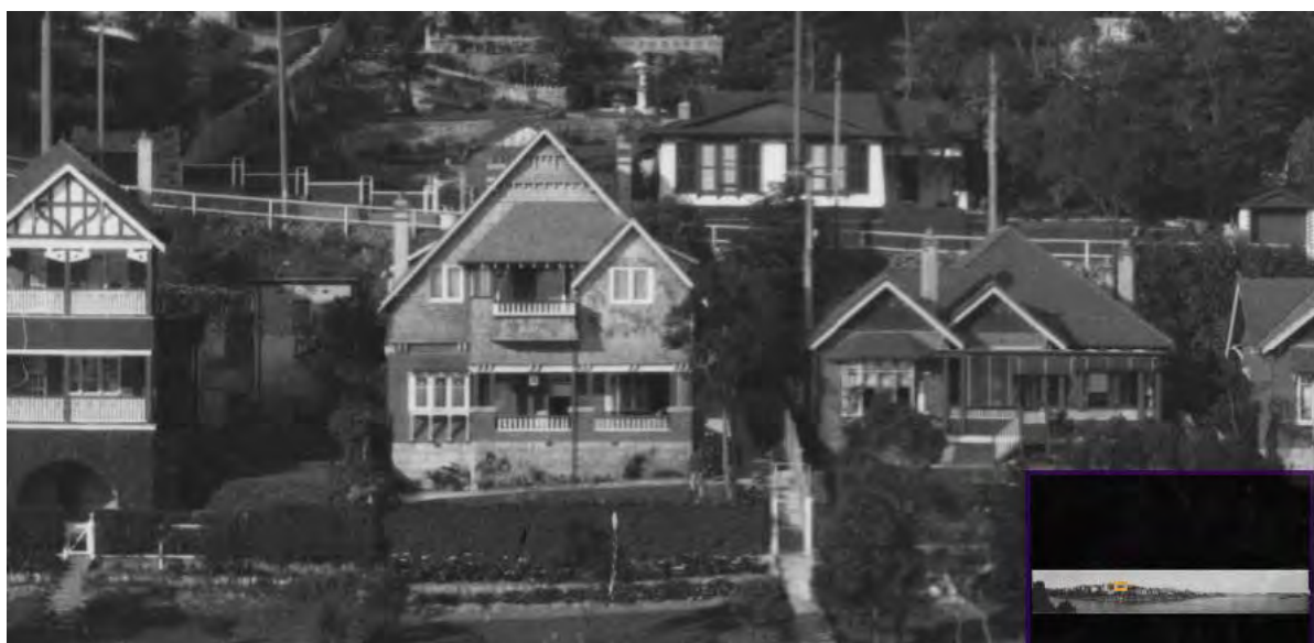
Figure 15: Excerpt from Panorama Cremorne Point c1921-1922: Trove: https://nla.gov.au/nla.obj-162273190/ Showing the original waterfront façade
