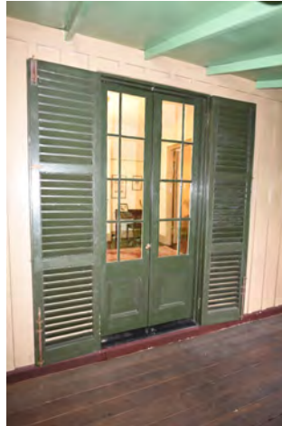
Figure 3. 27: Example of an original French door.
