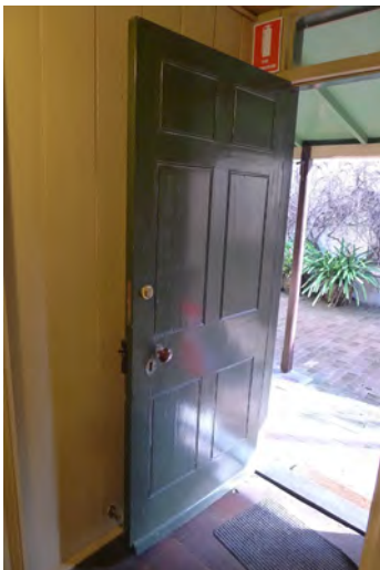
Figure 3. 72: Front door D01
