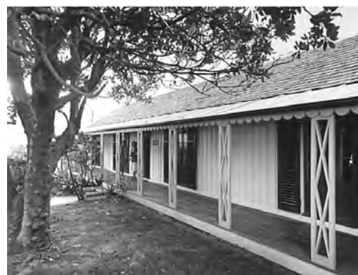
Figure 2. 51: Don Bank shortly after the completion of restoration works. Source: Stanton Library
