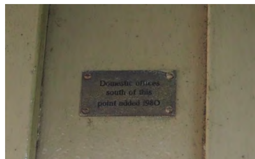
Figure 3. 63: A small plaque indicating extent of later works.
