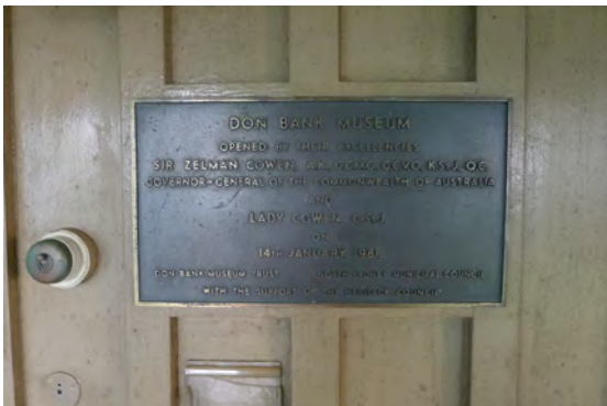
Figure 3. 60: Plaque located on front elevation adjacent to front door commemorating the opening of the Don Bank Museum.
