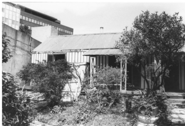
Figure 2. 41: Southern end of the front elevation of Don Bank prior to restoration works in c.1975. Courtesy: G. Britton
