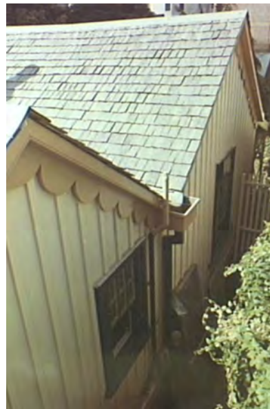
Figure 2. 49: The restored roofing of shingles. Source: Stanton Library (CPF 324)
