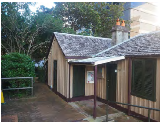
Figure 3. 18: North elevation of the house with adjacent paving and driveway leading to Oak Street.
