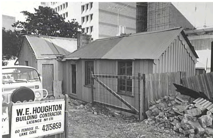
Figure 2. 46: The rear wing of Don Bank during restoration works c.1980. Source: Stanton Library (PF 2420)
