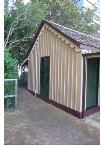
Figure 3. 28: North elevation of cottage.
