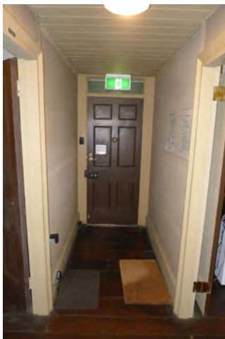
Figure 3. 44: Space 01, looking east towards front door
