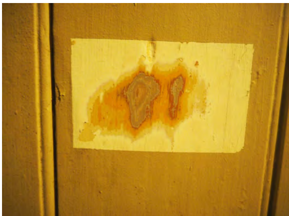
Figure 3. 64: Retained area in Space 02 showing results of paint scrapes.
