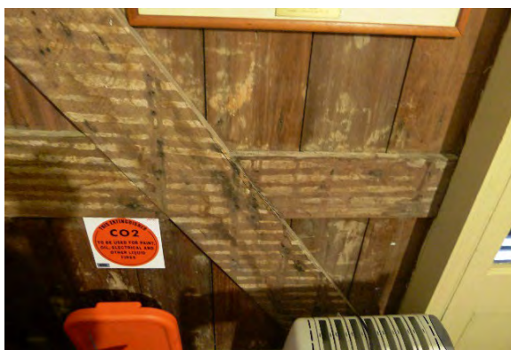
Figure 3. 71: Rails and boards in Space 03 with butt joints and evidence of lath and plaster.
