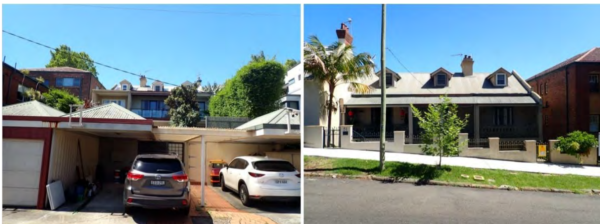
Figures 3 & 4 – Photo of subject site from the rear Commodore Street (left) and photo of front elevation from Union Street
