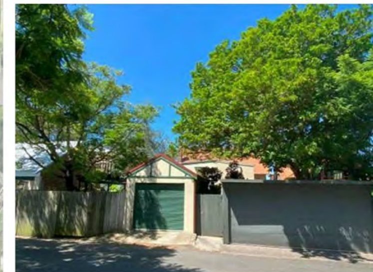
Rear Cremorne Lane view of 36 Cremorne Road, Cremorne Point.
