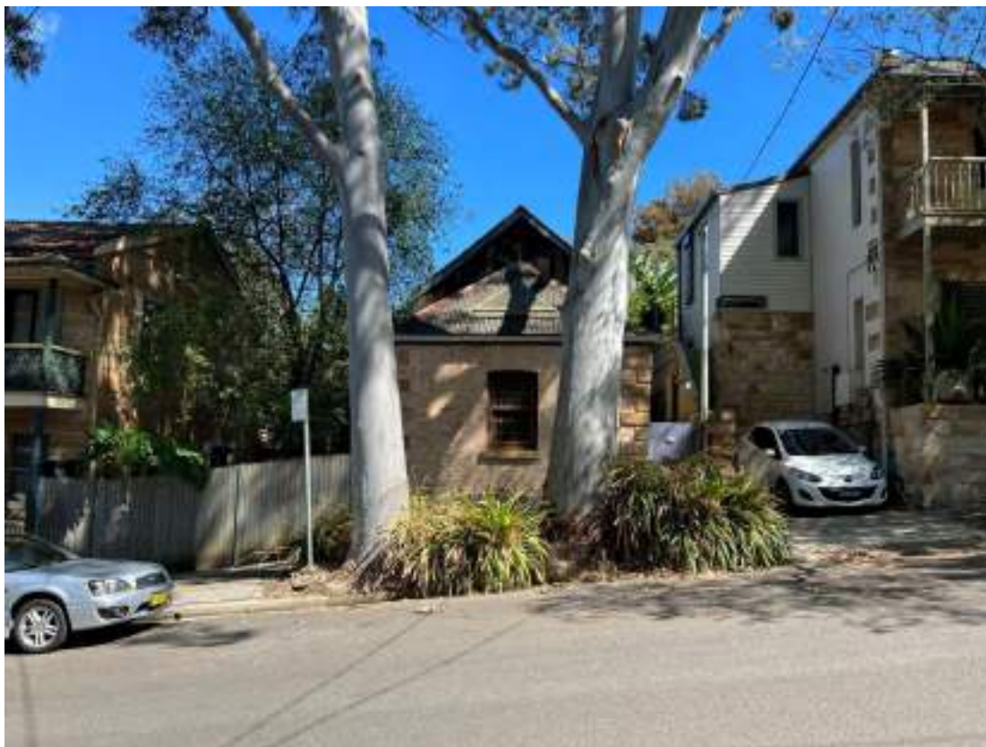
Subject place from opposite Euroka Street.
