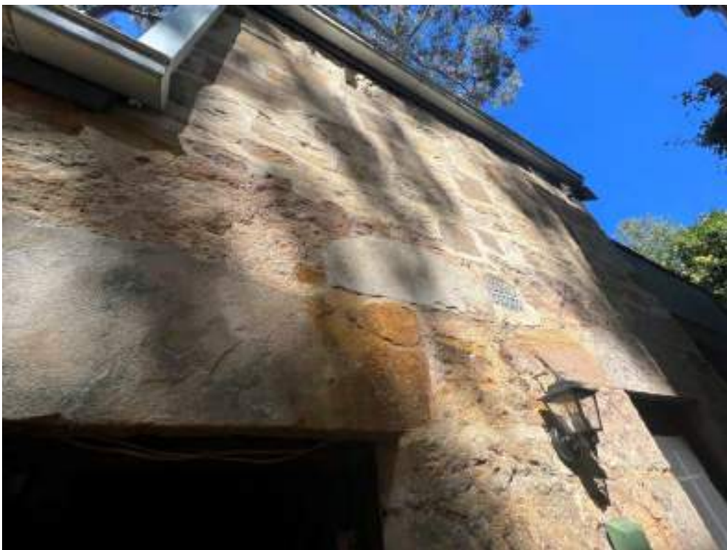
View to the sandstone wall of the loft addition, north elevation.
