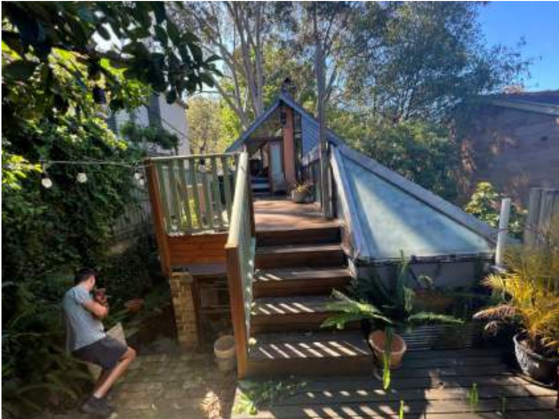
View from the backyard across the rear deck, which 'cuts' into the rear section of hip roof—all part of the 1980s redevelopment.
