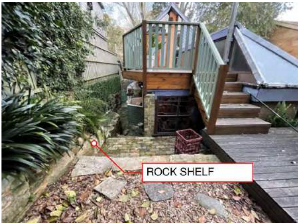
Figure 6- Photograph location C
