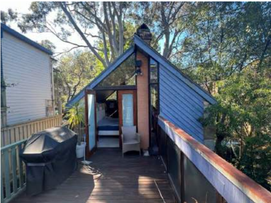
Rear elevation of the loft addition, showing the extended brick chimney.
