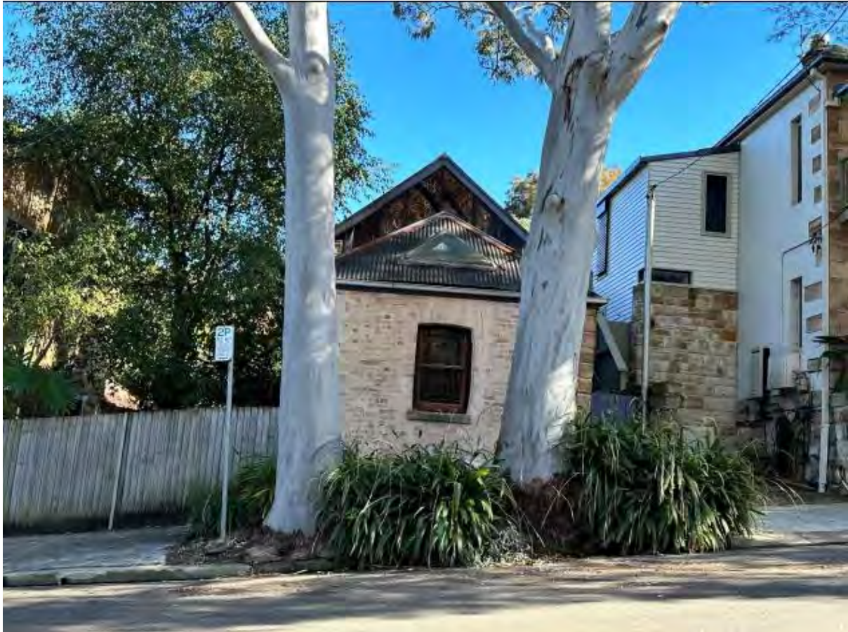
Figure 12: Front setback of subject site showing dwelling house and significant canopy trees (Blue Gum) in road reserve.
