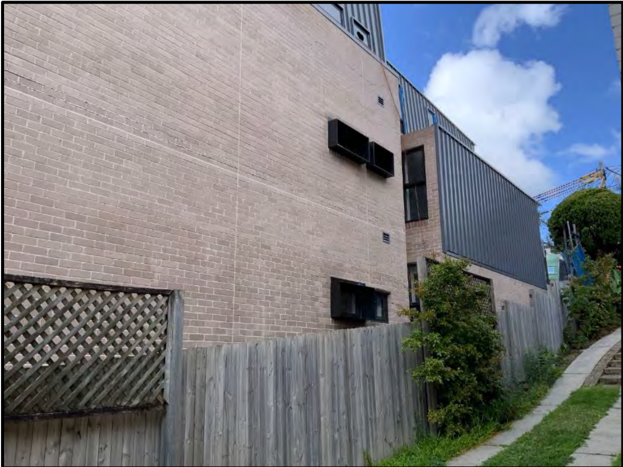
Figure 7: Photo of the southwestern elevation of the residential flat building under construction at 18 Illiliwa Street, noting the lack of openings, which avoids any visual bulk impacts associated with the height variation.
