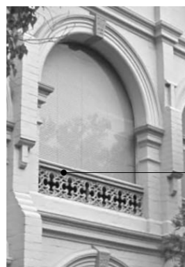
B1 - REINSTATE CAST IRON BALUSTRADE IN KEEPING WITH NO. 34 JEFFREY'S STREET
