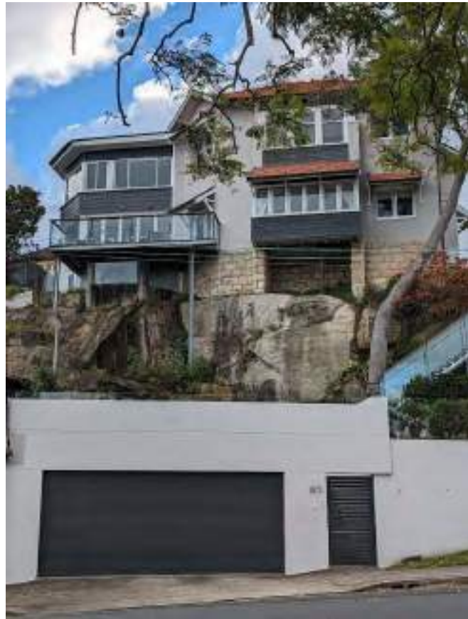
Existing Dwelling from Shellcove Road
