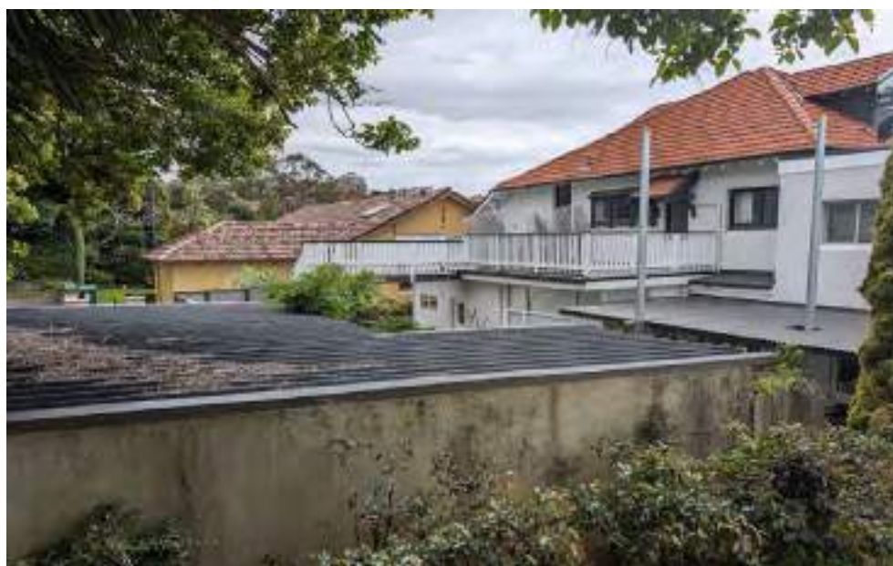
View of the rear of the subject dwelling from the rear ground floor verandah of No 53 Wycombe Road. To the right the southwestern corners of the extension, represented by the metal poles (parapet on the edge of a proposed flat roof), is indicated. In the centre and to the left of the image is the deck and stairway being partly replaced by the extension, the stairs being replaced by a new staircase inside the house, accessing all levels, including the attic. In the foreground is the roof and southern wall (close to or on the boundary) of the existing garage on the site.
