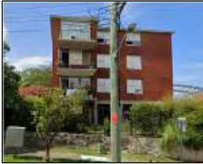
Figure 11: Existing western façade
