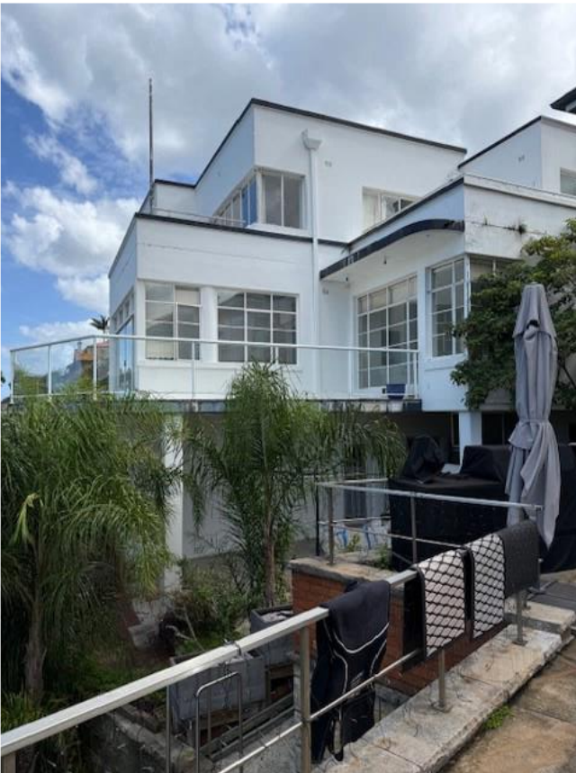
Photo 7: View from existing ground level terrace to the north towards 186 Kurraba Road
