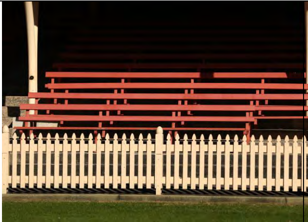
North Sydney Oval Picket Fence replacement 2015
