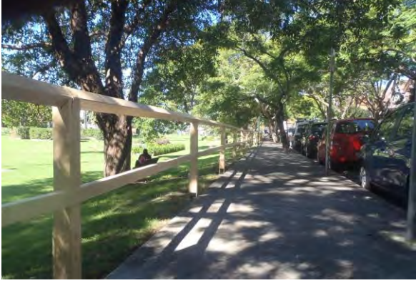
McDougall Street Kirribilli – Timber Fence replacement 2016
