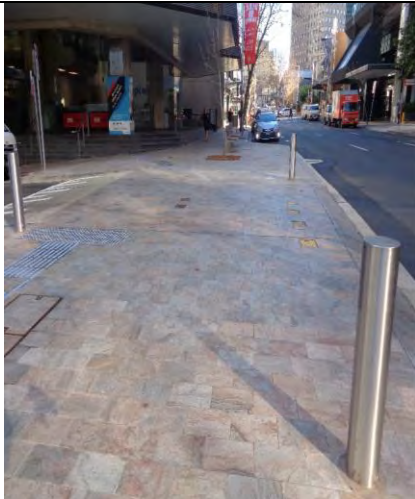
Berry Street new – stainless steel traffic bollards 2017
