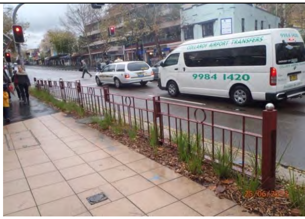
Military Road Neutral Bay (After) –Decorative Safety Fence
