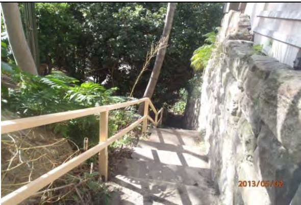
Doris Street – Neutral Bay – Fence Repairs 2015
