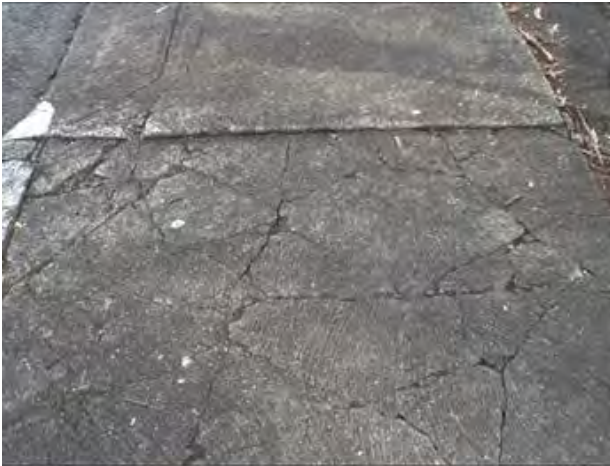
Concrete footpath in poor condition
