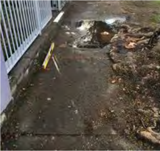
Tree root affected concrete footpath including ponding
