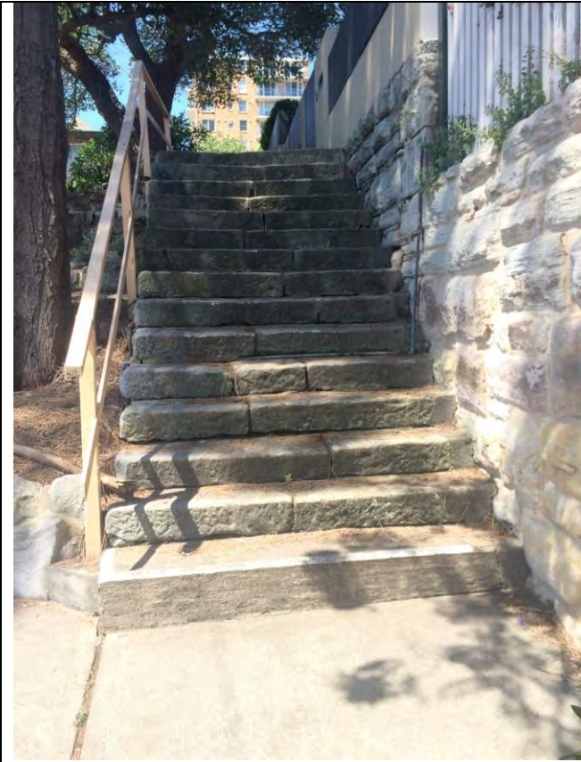
Stratford Road, Cammeray – Before
