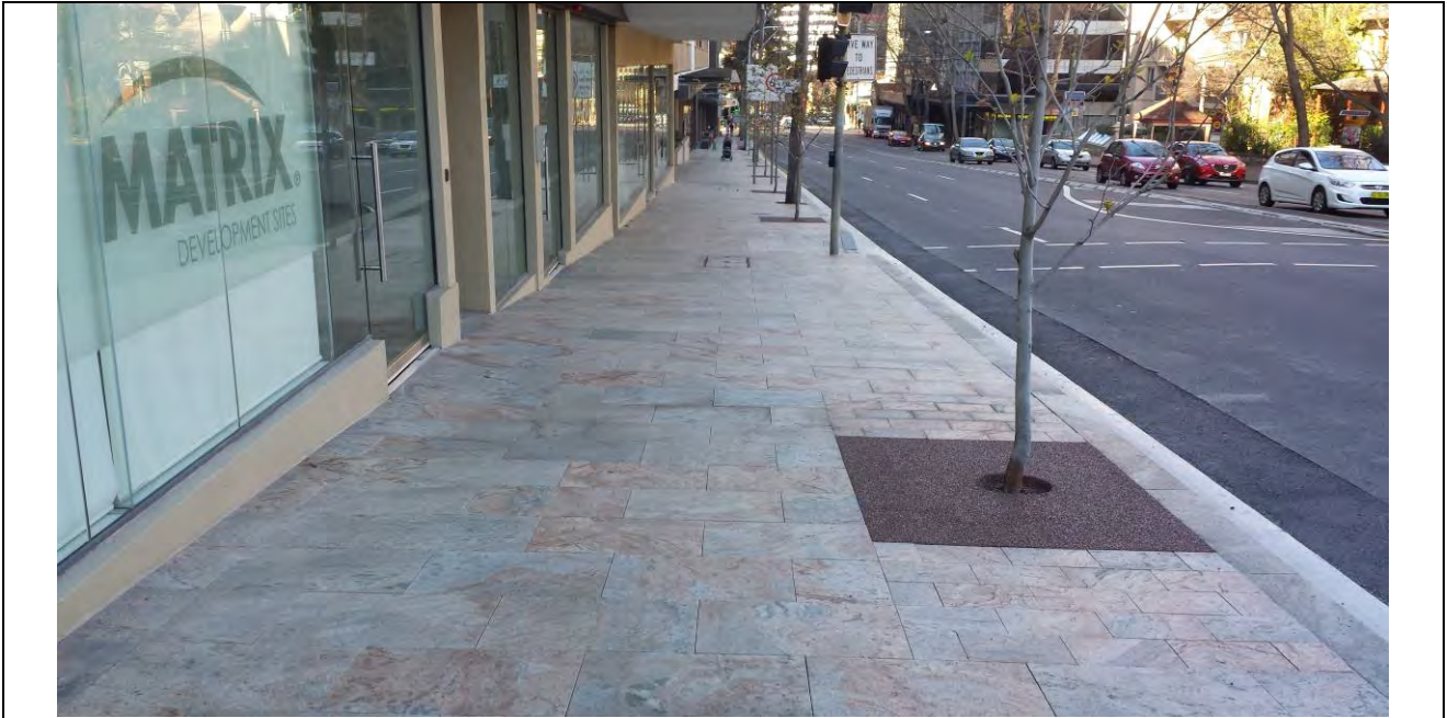
Pacific Highway, North Sydney – Granite
