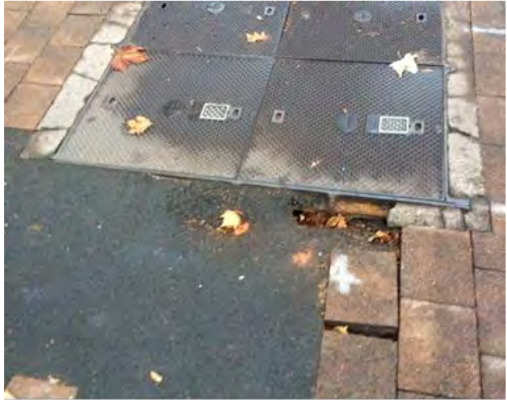
Footpath collapse due to base course wash out
