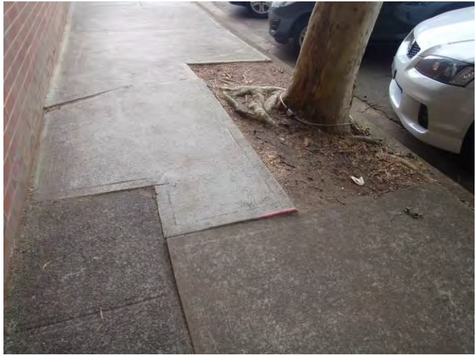
Tree root affected concrete footpath including ponding
