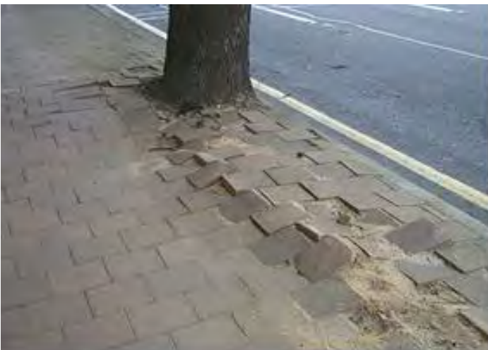
Tree root affected pavers and tree site infill
