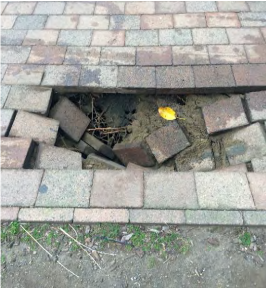
Footpath collapse due to base course wash out
