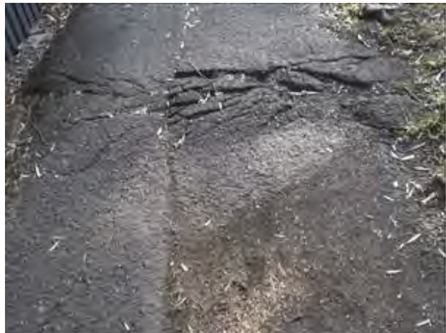
Asphaltic concrete footpath in poor condition
