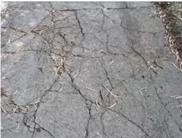
Asphaltic concrete footpath in poor condition
