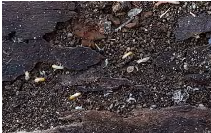
Termites found in timber marine structure
