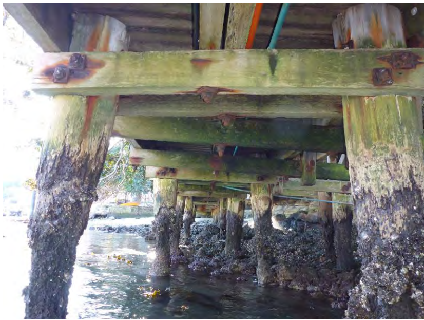
Examples timber piles – Hayes Street Boardwalk – Currently closed
