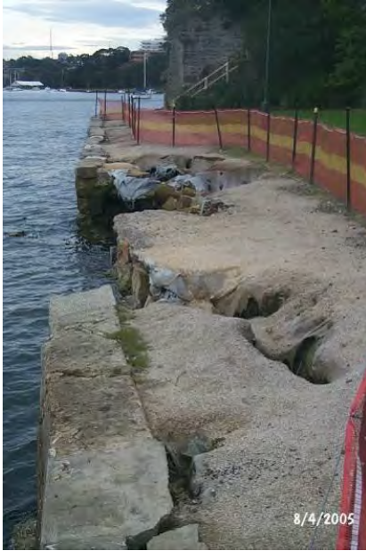
Examples of failed and failing seawalls in the North Sydney LGA – Blues Point
