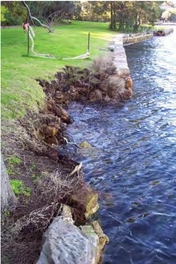
Examples of failed and failing seawalls in the North Sydney LGA – Sawmillers Reserve
