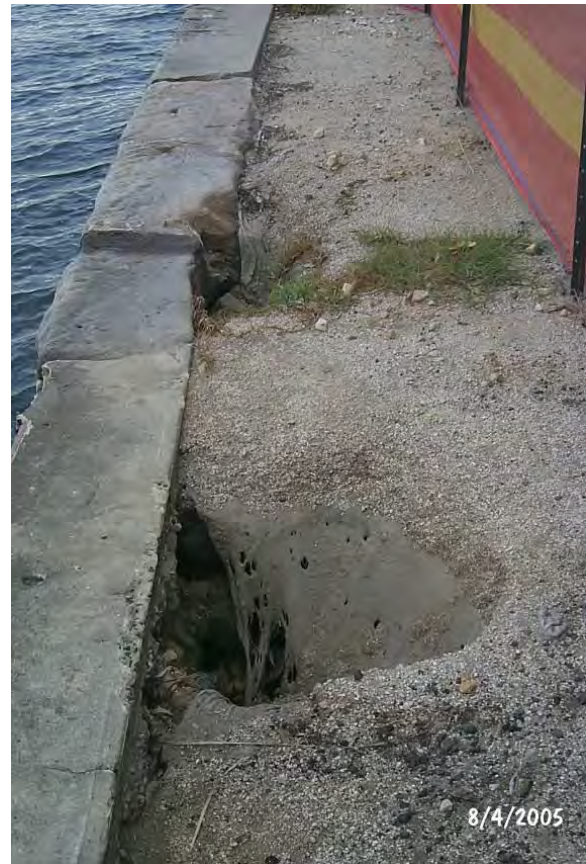
Examples of failed and failing seawalls in the North Sydney LGA – McMahon's Point
