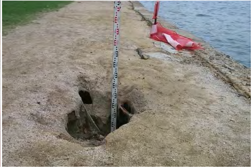
Examples of failed and failing seawalls in the North Sydney LGA – Blues Point
