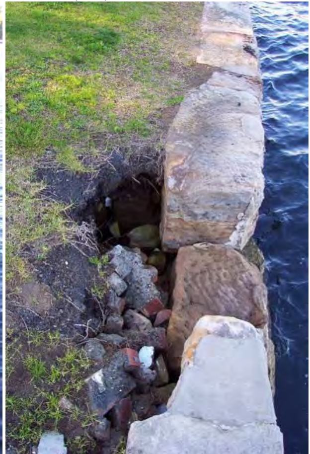
Examples of failed and failing seawalls in the North Sydney LGA – Sawmillers Reserve
