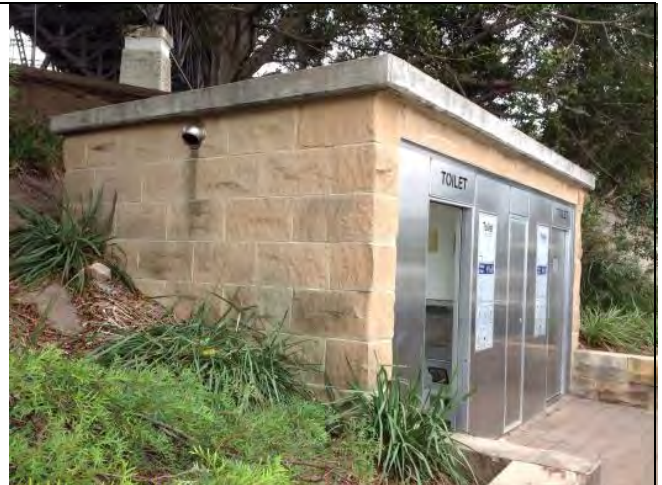
Bradfield Park – Exeloo Toilets
