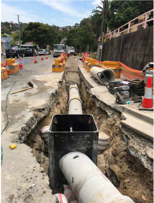
Pit and Pipe replacement at Milson Road, Cremorne Point.
