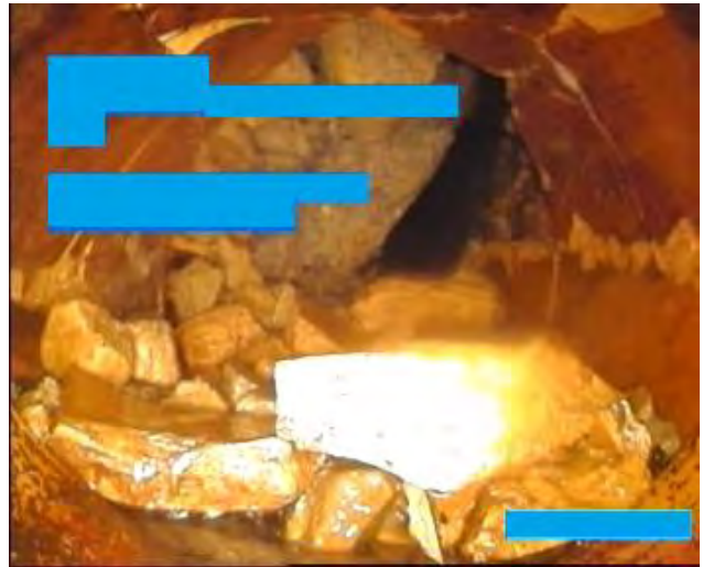
Stormwater Pipes in very poor condition – collapsed and blocked
