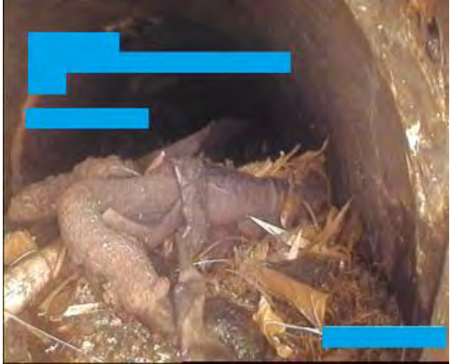
Stormwater Pipes in very poor condition – Tree root infiltrations and blocked
