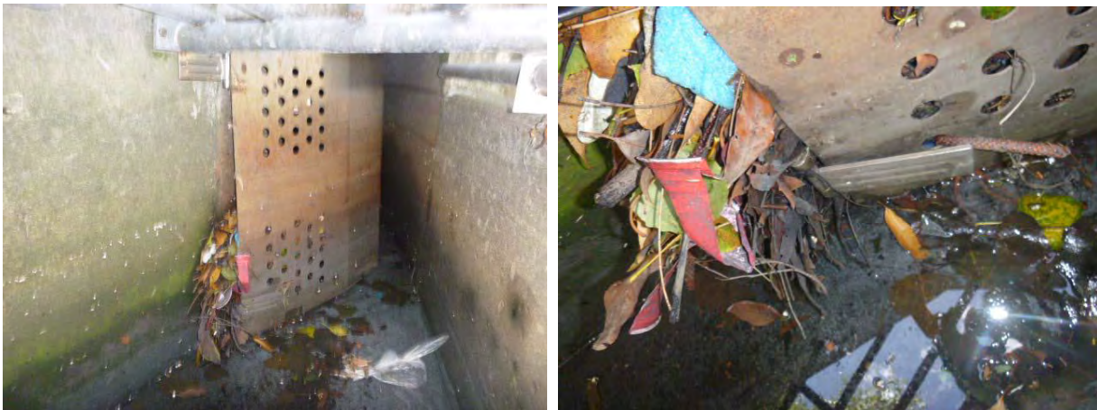
The floatables flap was jammed open due to a broken hinge and pollution trapped in it stopping it closing.
