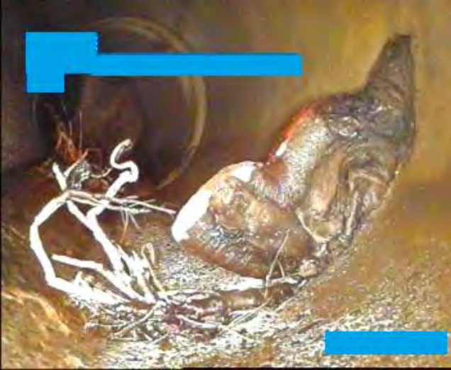
Stormwater Pipes in very poor condition – Tree root infiltrations and blocked
