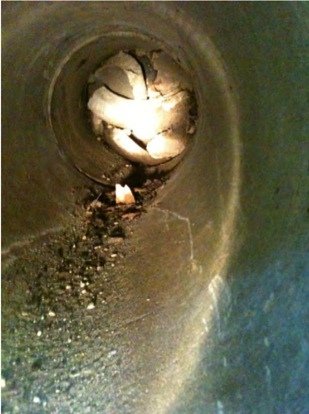
Stormwater Pipes in very poor condition – collapsed and blocked
