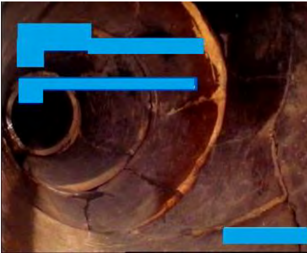
Stormwater Pipes in very poor condition – collapsed and blocked
