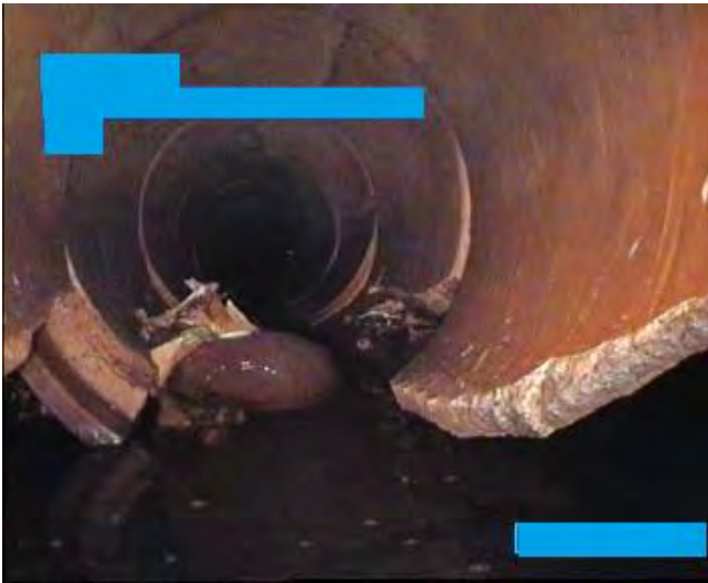
Stormwater Pipes in very poor condition – collapsed
