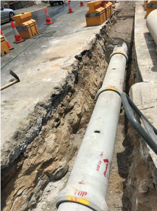
Pit and Pipe replacement at Milson Road, Cremorne Point.
