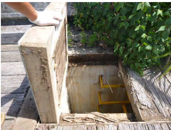
Lids are too heavy - The wood is starting to chip; they should be replaced. Lifting points rusted or broken off
