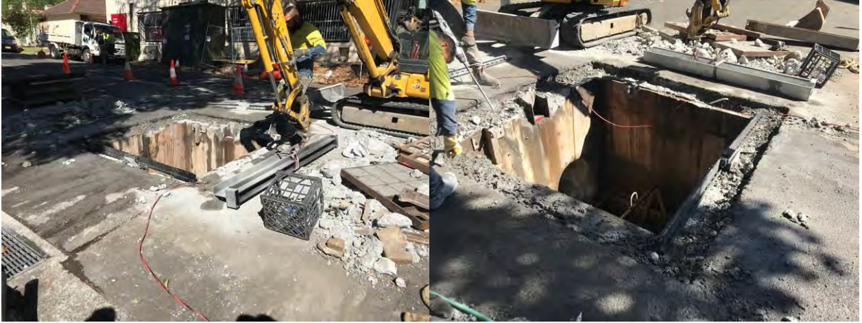
Replacement of GPT Lids at Elamang Avenue, Neutral Bay.
