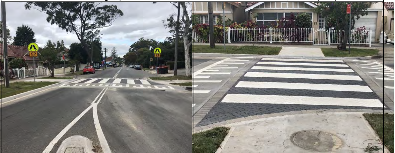
Pedestrian Crossing Upgrade – Spofforth Street, Cremorne
