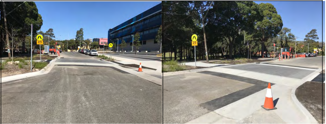
Pedestrian Crossing – Anzac Avenue, Cammeray
