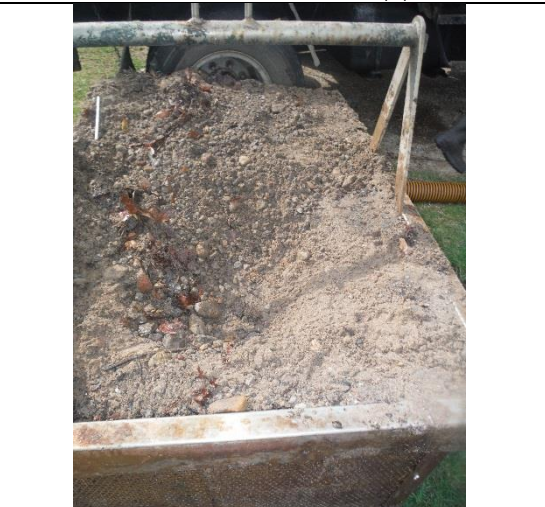
Litter Basket full of silt prior to cleaning
