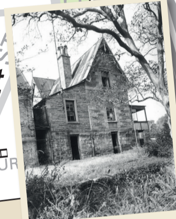
Address shortly before demolition 1958
