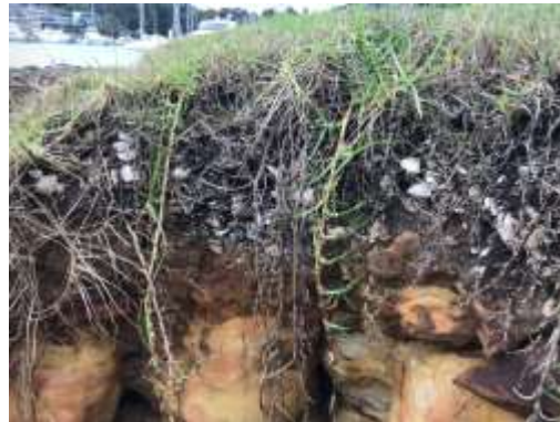
Coastal erosion monitoring, Bayview
