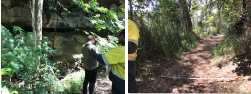
Track upgrades, East Lindfield
