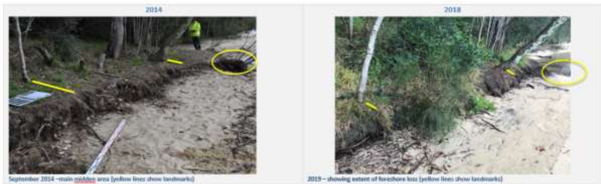
Coastal Erosion between 2014 and 2018, Middle Harbour
