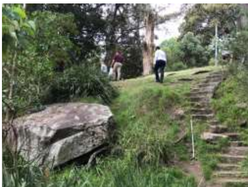
Stair upgrade, Waverton
