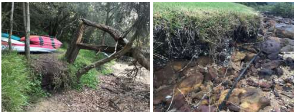
Monitoring confirms ongoing impacts due to coastal erosion
