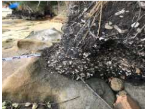
Coastal erosion monitoring, Northbridge
