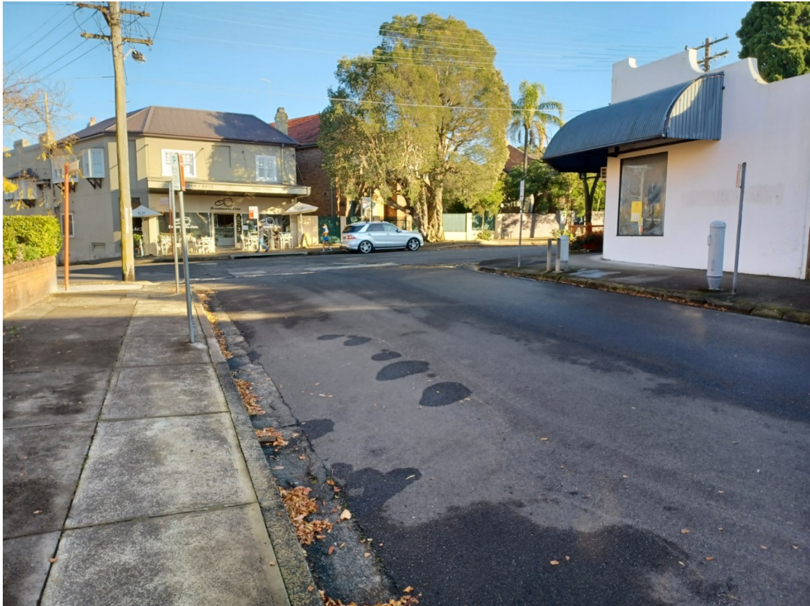
Photo 3. The existing site – 21/06/22
