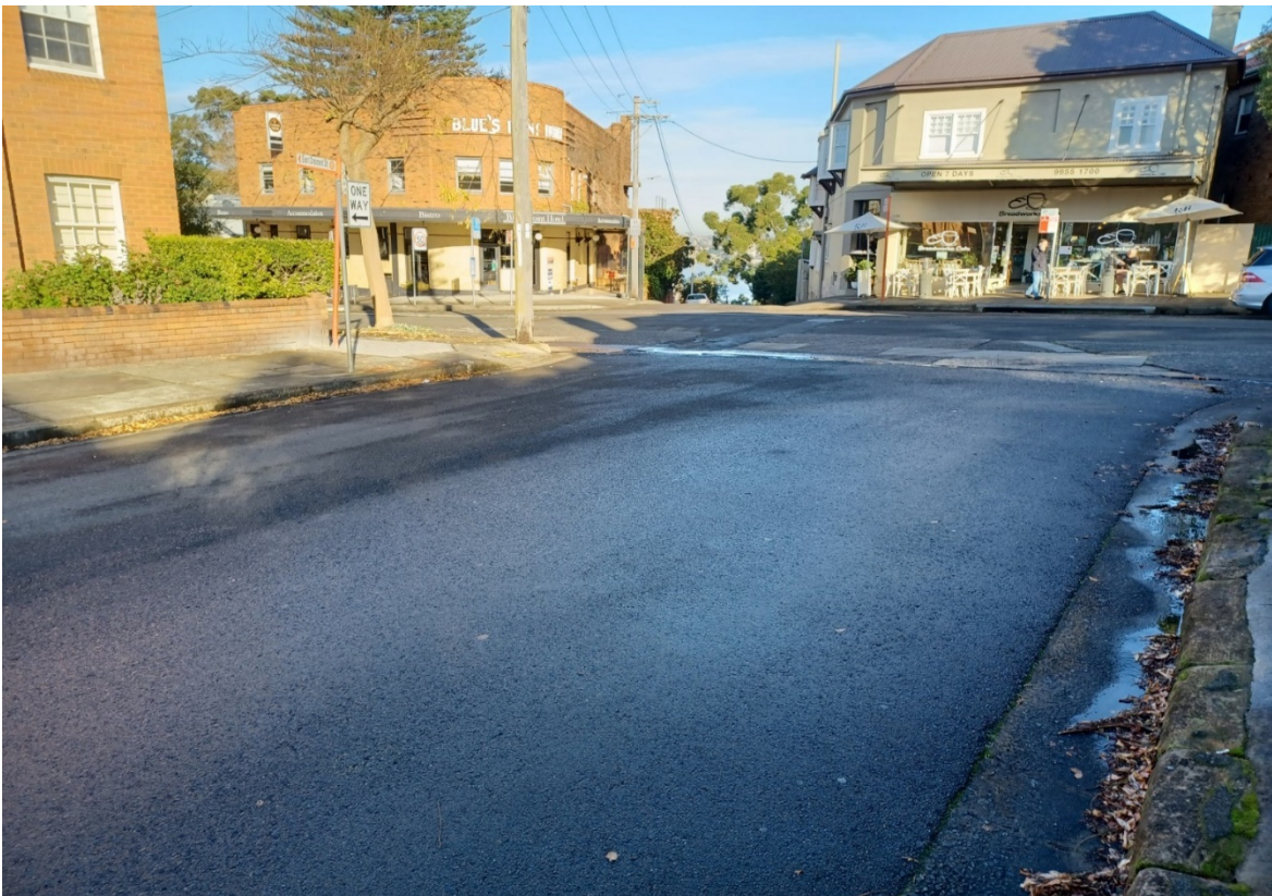
Photo 4. The existing site – 21/06/22
