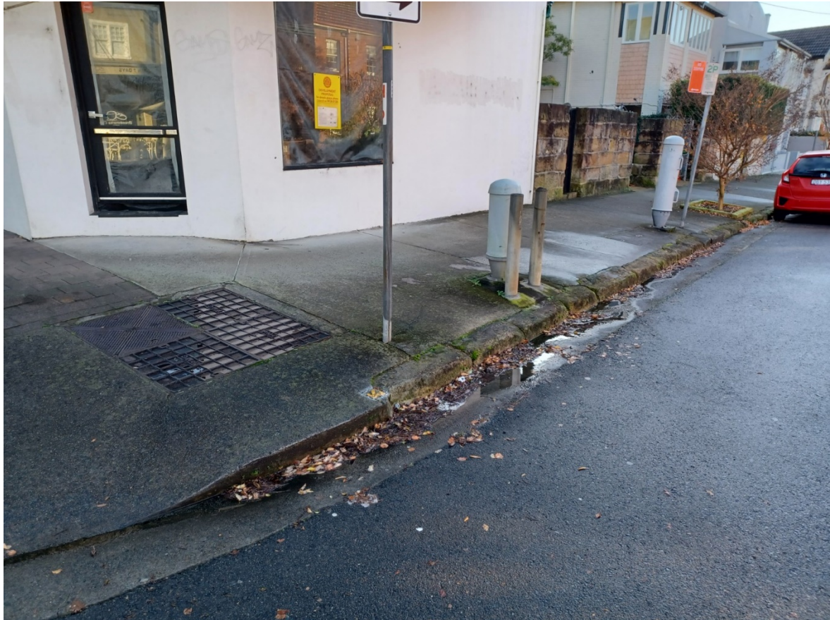
Photo 5. The existing site – 21/06/22
