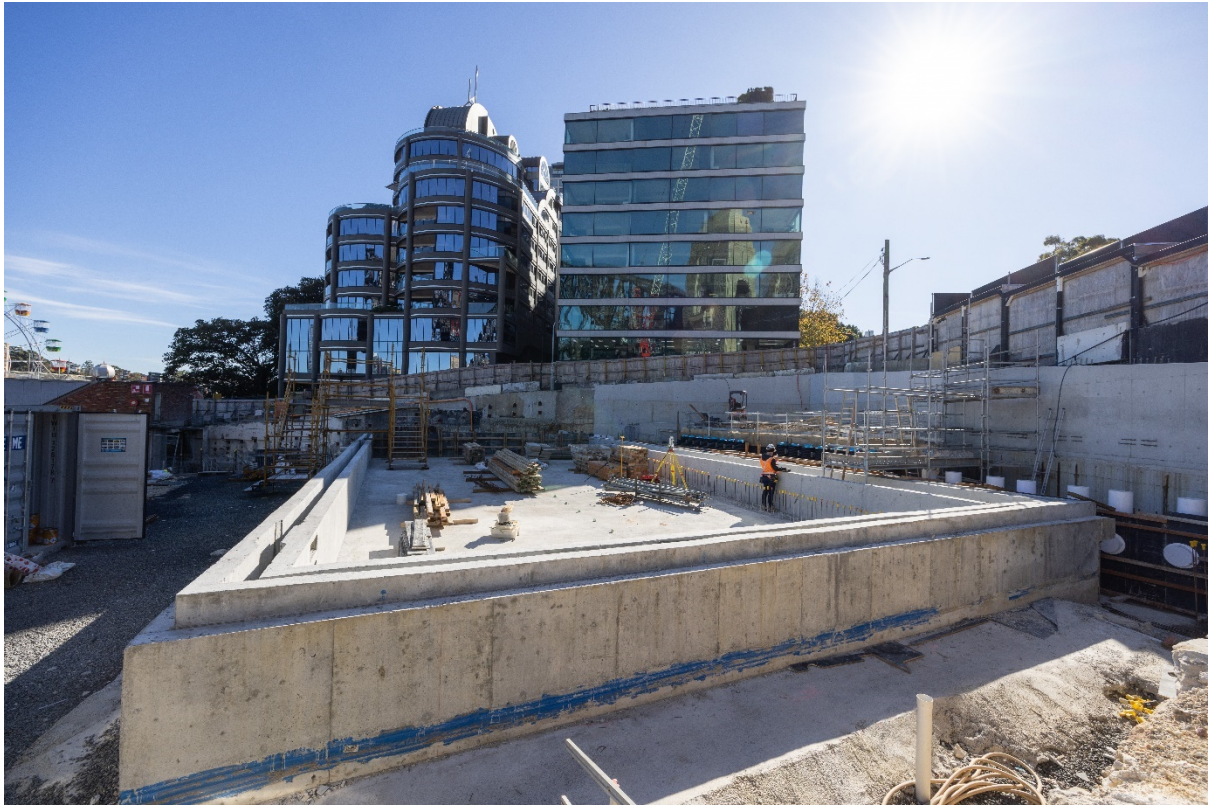
Program pool under construction 09/06/2022
