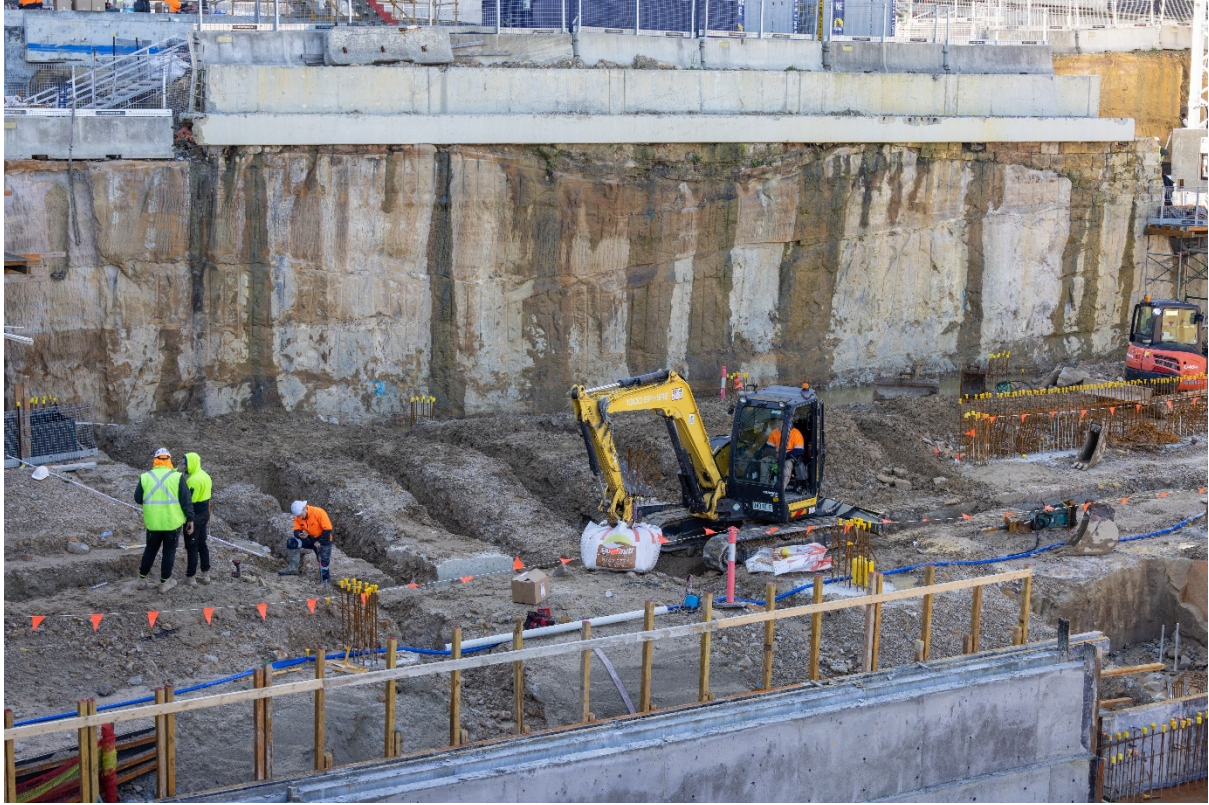
Grandstand inground services underway 08/07/2022
