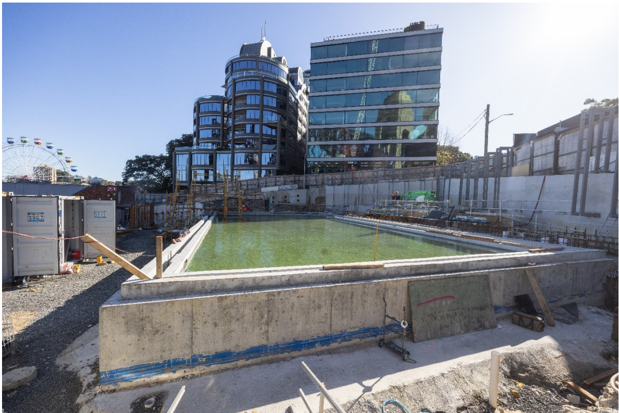
Program pool leak testing under way 08/07/2022
