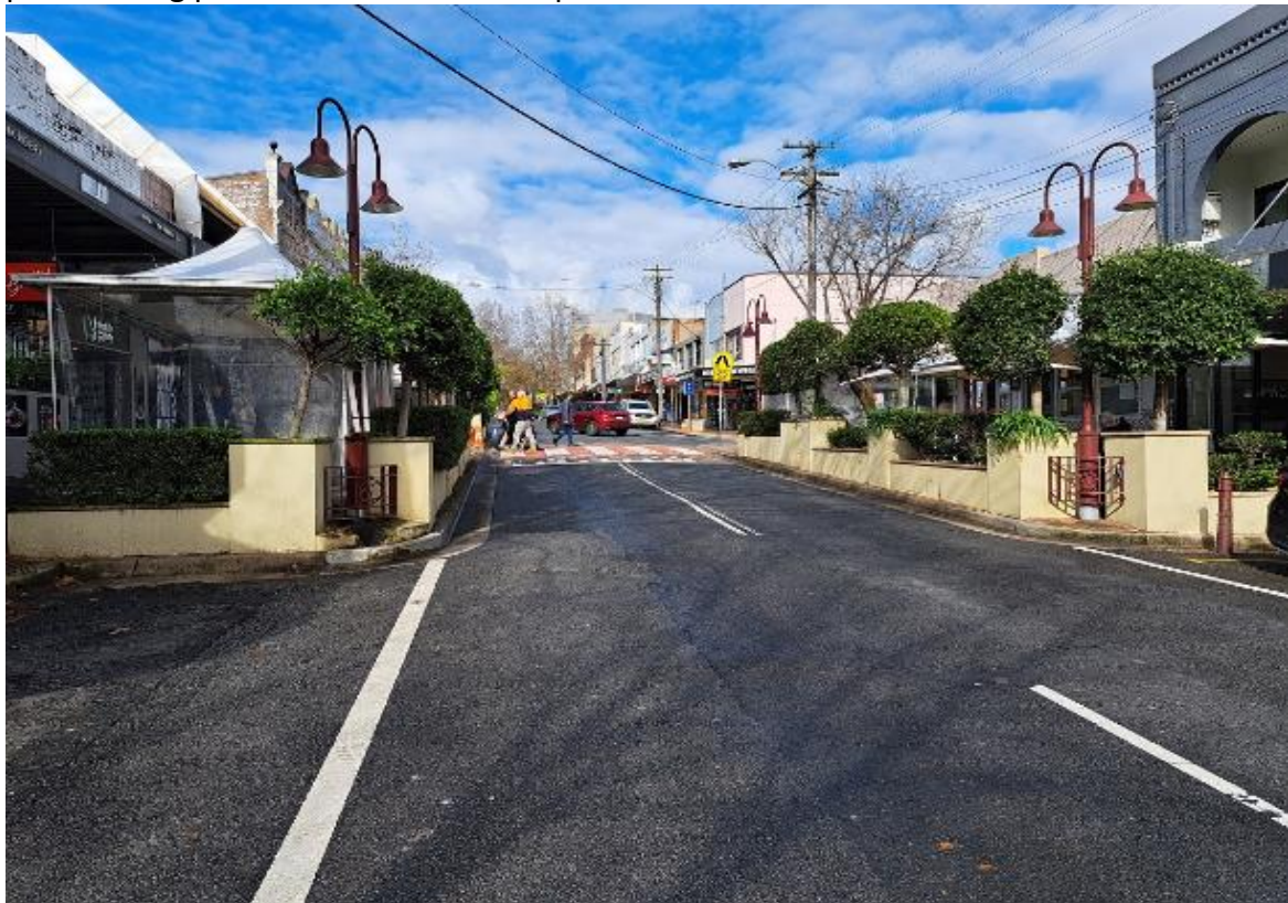
Photo 9. Stage 2 Willoughby Road upgrade facing Clarke Street– old 'Goose Neck' lights & planter boxes to be updated
