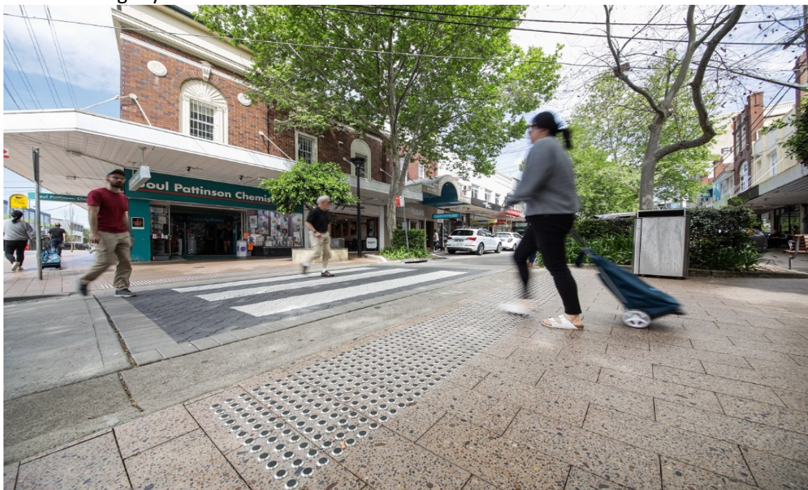
Photo 1. Photo of Stage 1 of Willoughby Road upgrade, completed in 2019 showing new raised pedestrian crossing
