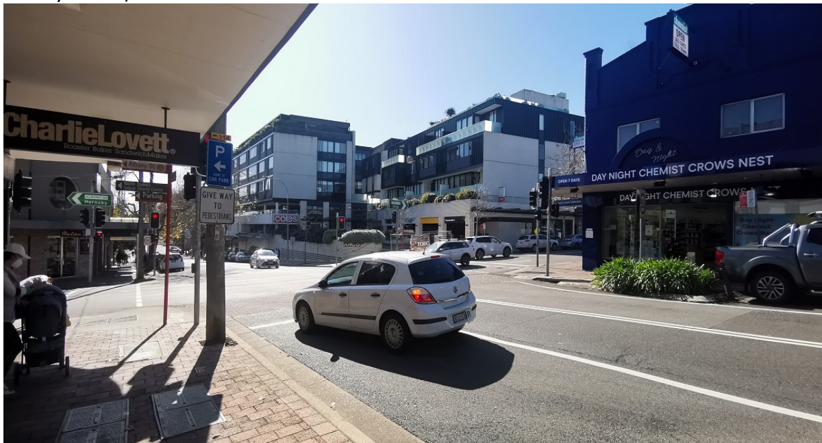
Photo 6. Photo showing the end of Stage 2 Willoughby Road Upgrade at the intersection of Albany Street - Existing
