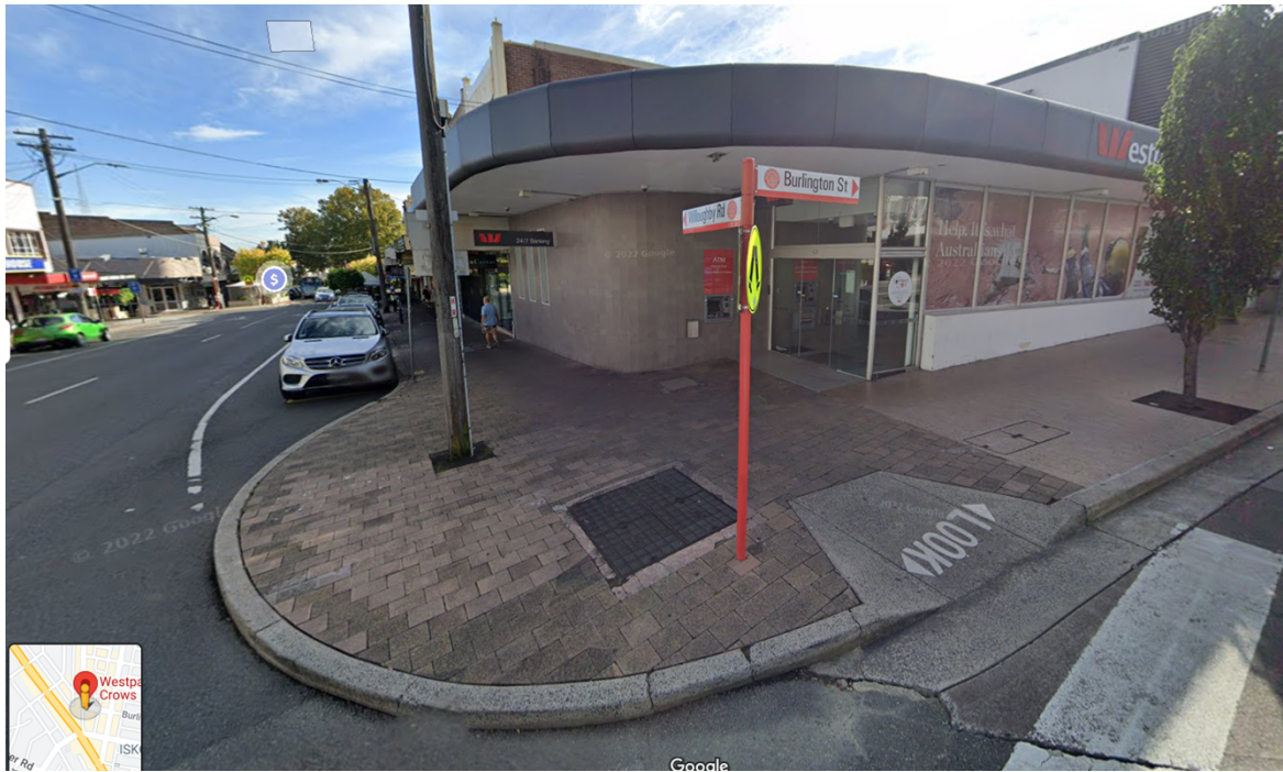
Photo 5. Photo showing start of stage 2 Willoughby Road upgrade, corner Burlington Street – Existing
