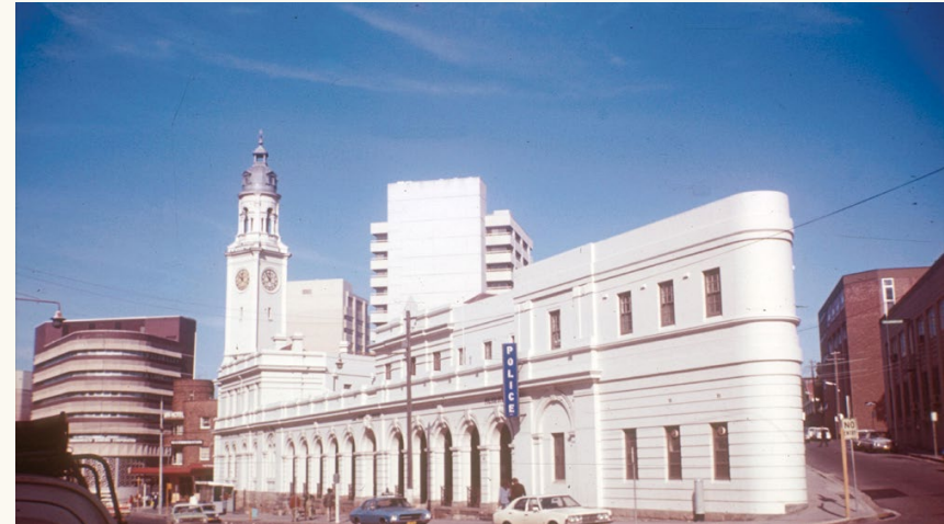
The North Sydney Post Office, Courthouse and Police Station complex in 1974. Stanton Library collection.
