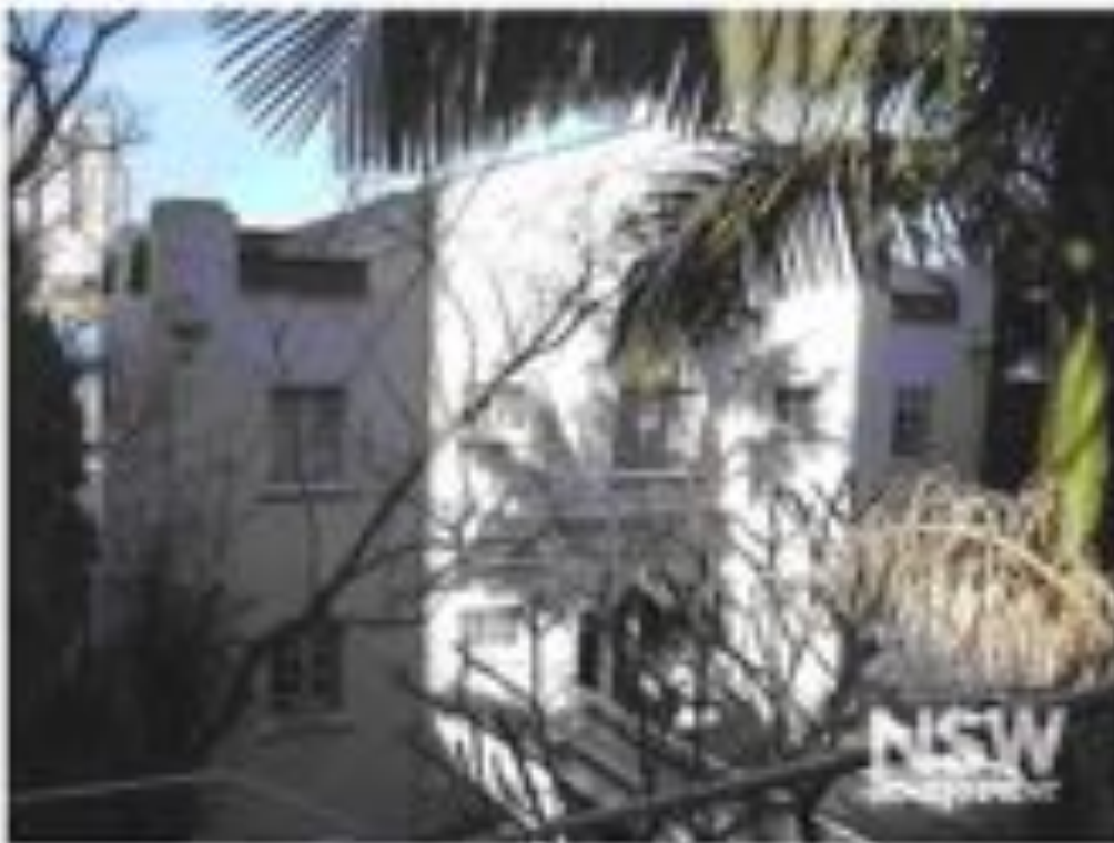
19 East Crescent Street, McMahons Point. Source: Heritage NSW SHI form
