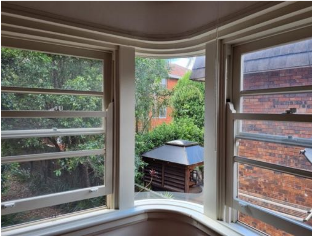
Figure 16: Curved glass to corner, with typical timber framed double hung windows with horizontal glazing bars to either side. Source: photo supplied by North Sydney Council
