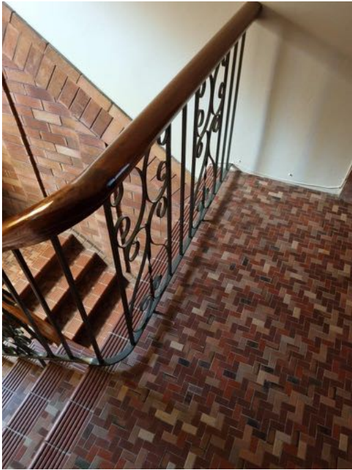
Figure 14: (Left) stairwell, showing more detail of original tiling Source: photo supplied by North Sydney Council
