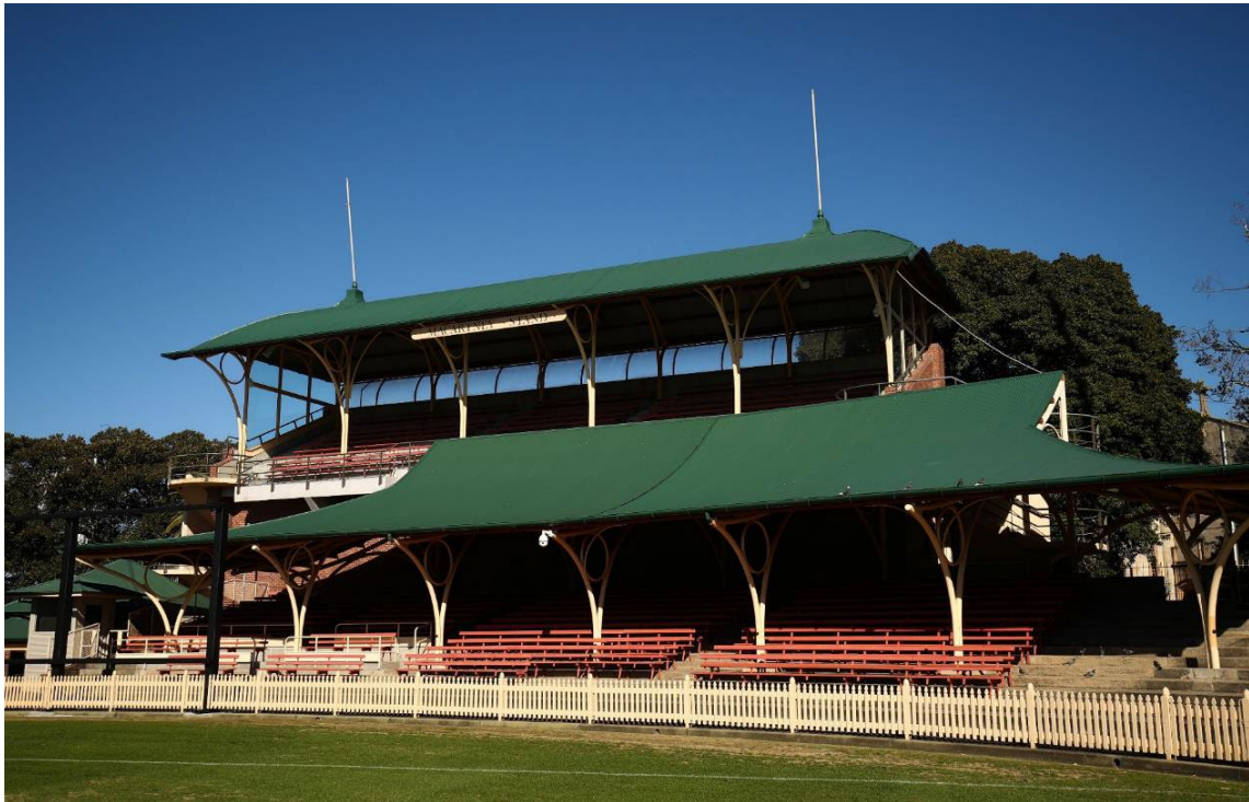
Councils Property team organise and undertake significant maintenance works on North Sydney Oval including roof replacement of the grandstands- painting and structural repairs each year.
