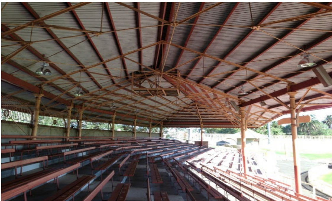
Councils Property team organise and undertake significant maintenance works on North Sydney Oval including roof replacement of the grandstands- painting and structural repairs each year
