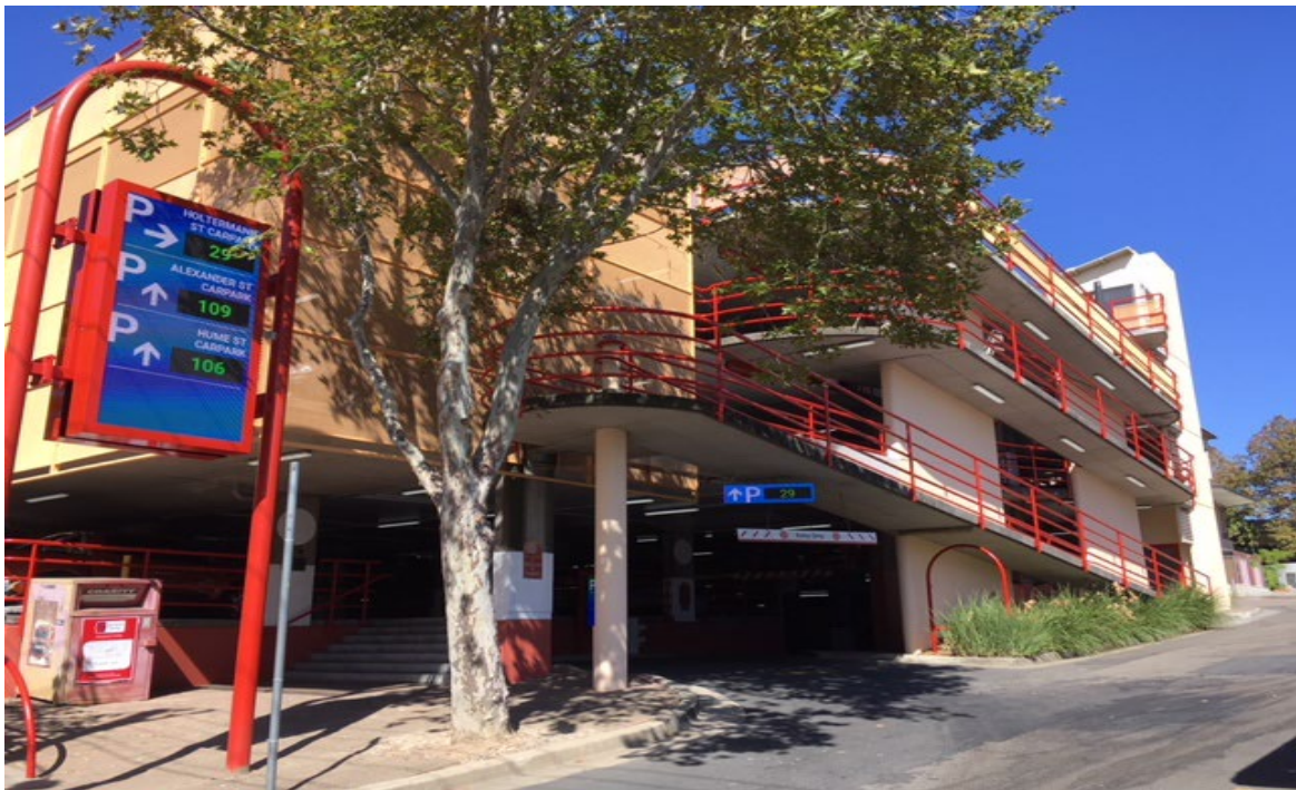
Holtermann Street Car park Redevelopment – undergrounding the carpark and construction of a roof top park. Project includes the architectural treatment of the Northern façade of the Crows Nest Center. Currently in design – Existing Carpark.
