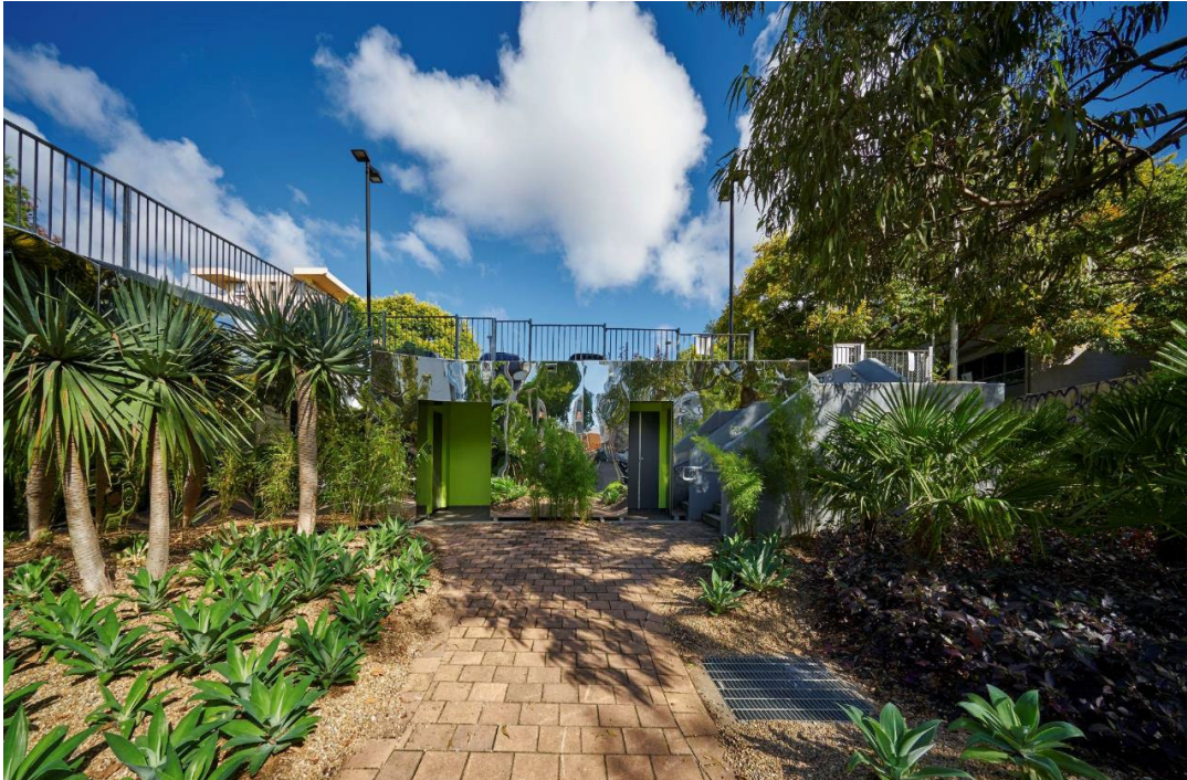
New Public Toilets have been built in the Barry Street Carpark – Neutral Bay in 2016 – costs $450K
