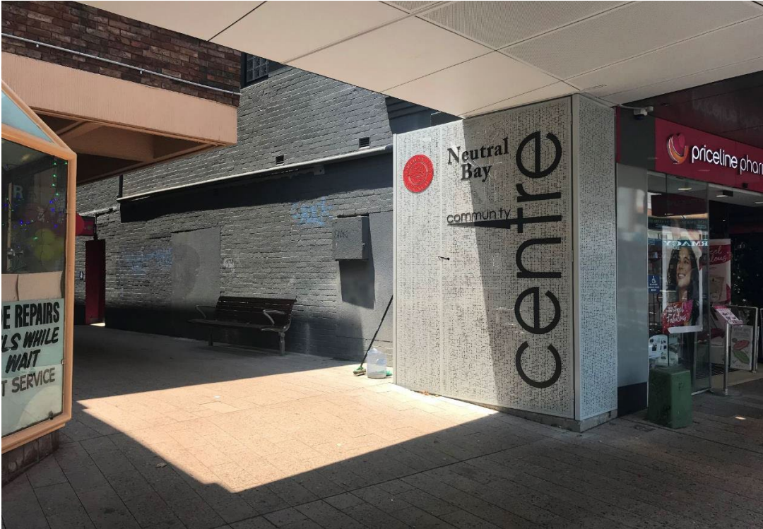
Upgrade of the Neutral Bay Community Centre – completed April 2019
