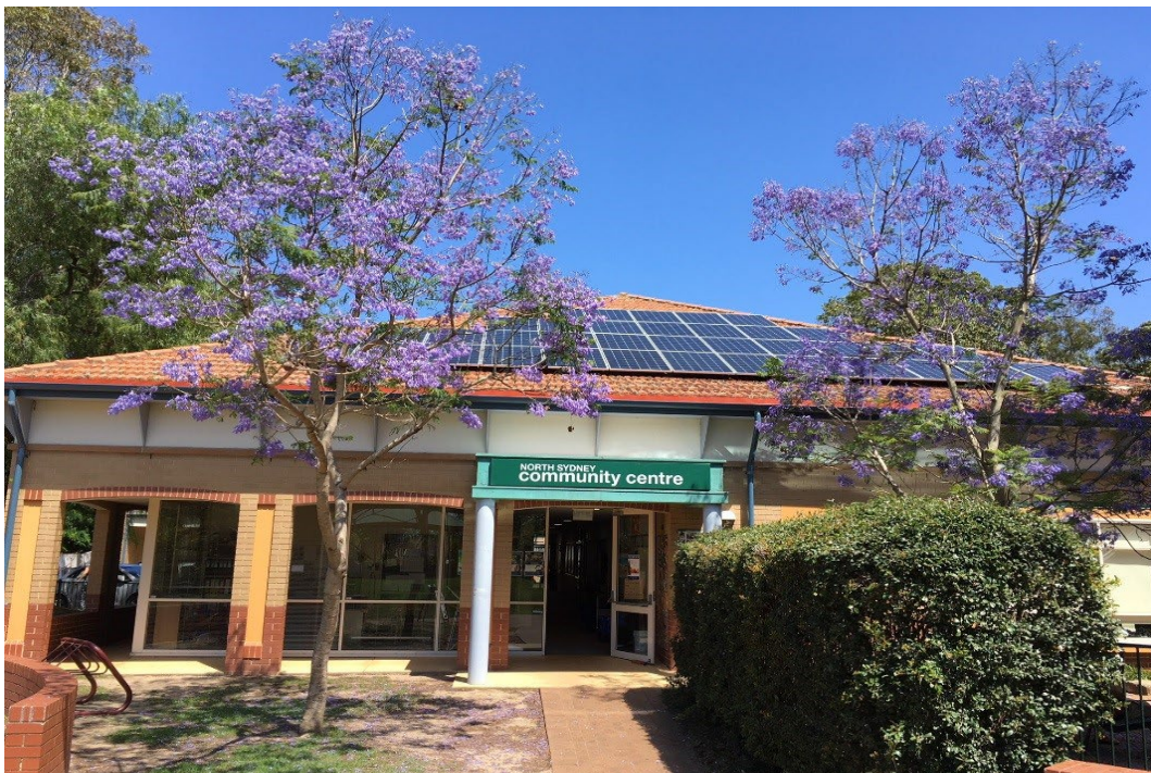
Solar Panels have been rolled out across a number of Councils Community and operational buildings over the last 5 years as part of an ongoing program. North Sydney Community Centre
