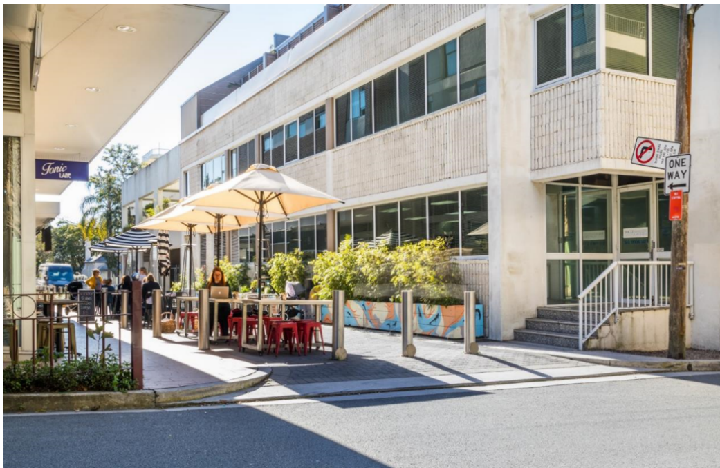
Young Lane Closure and Upgrade – completed in 2015
