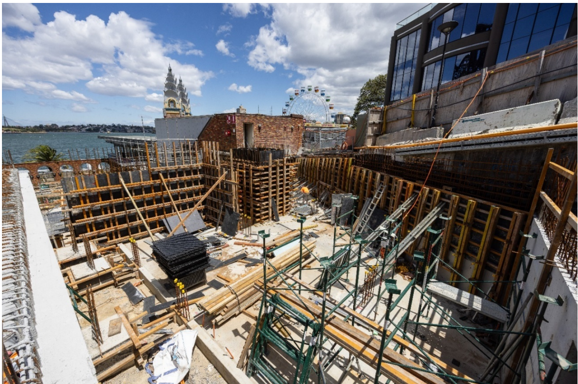
Level 2 plant room and Paul St retaining wall 21/11/2022
