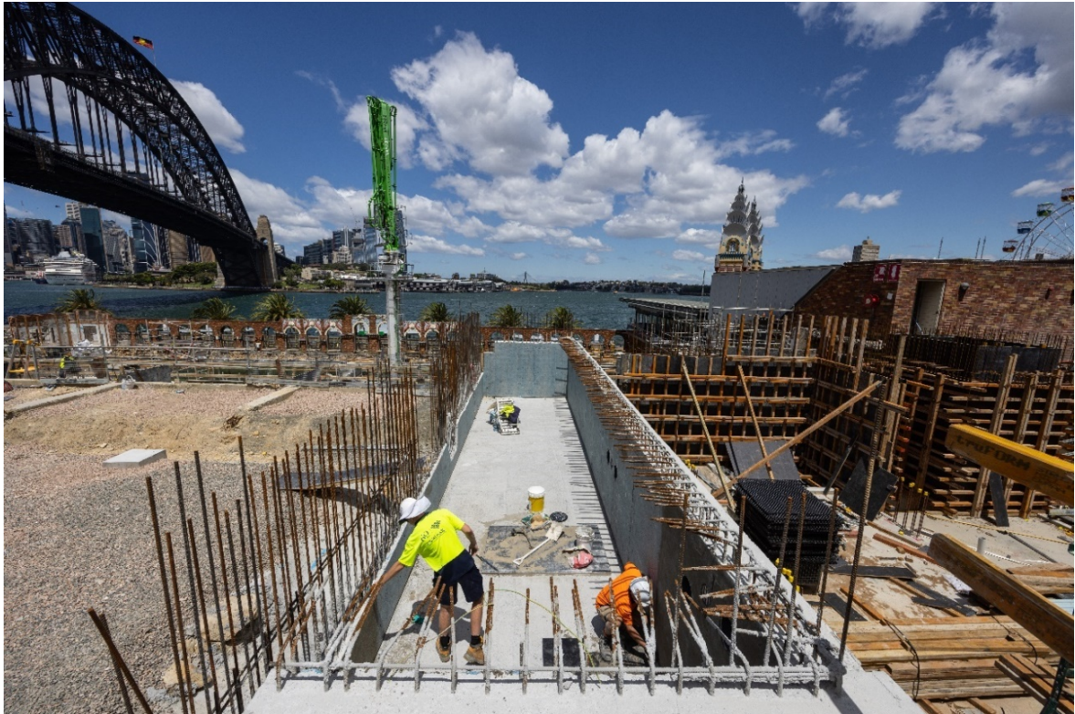
25m pool balance tank 21/11/2022
