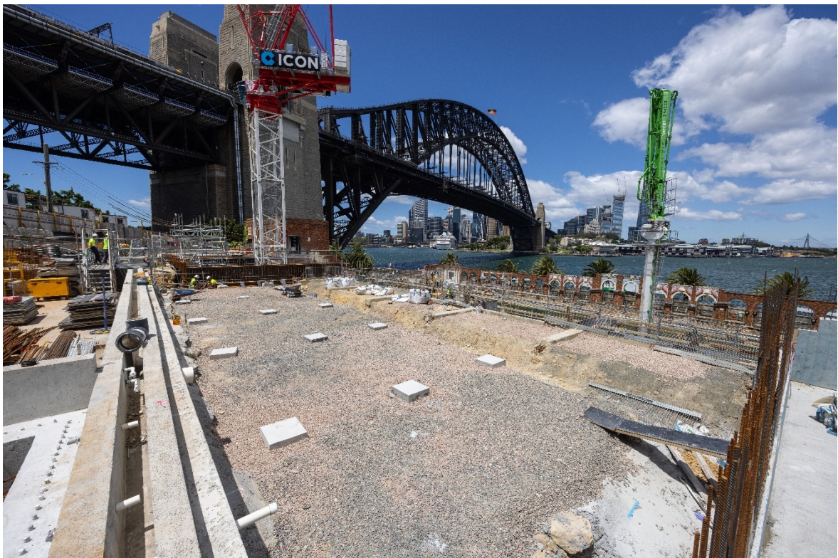
25m pool preparation commenced 21/11/2022
