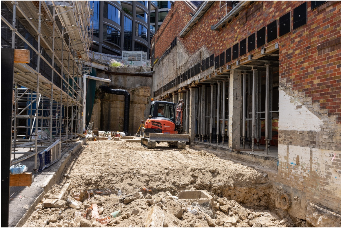
Western Stairs slab preparation 21/11/2022
