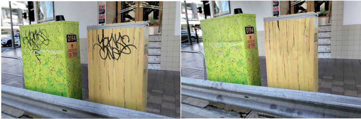
Before and After photos of typical Instance of Graffiti in North Sydney on the RMS Control box – Military Road, Neutral Bay
