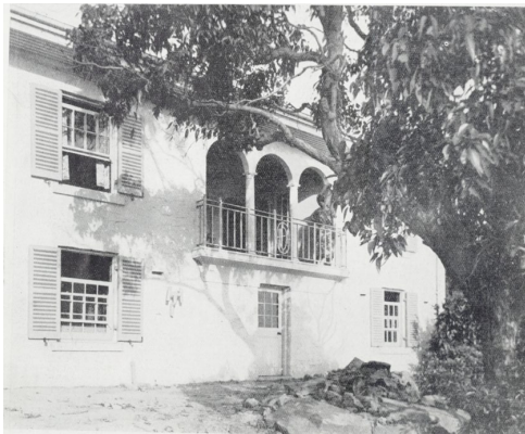
Figure 2. 8: The east (harbour front) elevation of Nutcote. Photograph by H. Cazneau. Source: The Australian Home Beautiful , March 12, 1926
