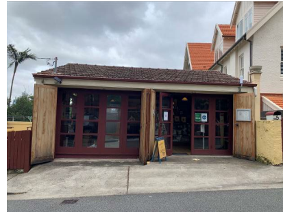
Figure 3. 111: Street elevation of the Garage
