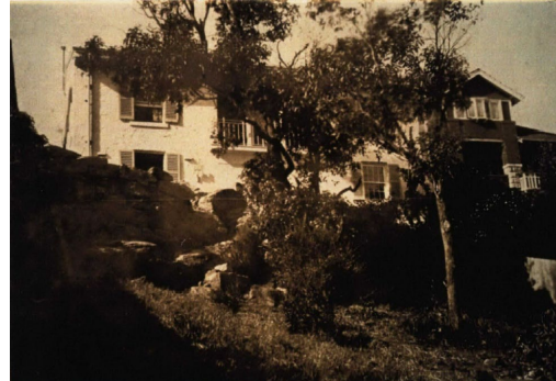
Figure 2. 25: 1930s view of the harbour front garden and Nutcote. Source: Nutcote CMP 1993, p. 29
