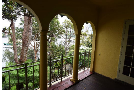
Figure 3. 95: Loggia with door from Dining Room
