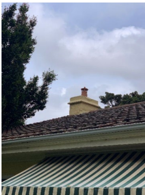
Figure 3. 64: Chimney and roof pan tiles
