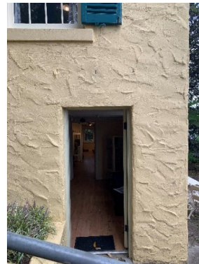
Figure 3. 73: Entry into former Laundry in the lower level
