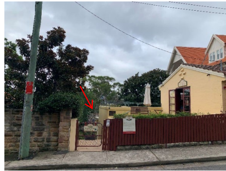
Figure 3. 7: Glimpse view V12 of the roof of the Main House seen through entry gate from Wallaringa Avenue.
