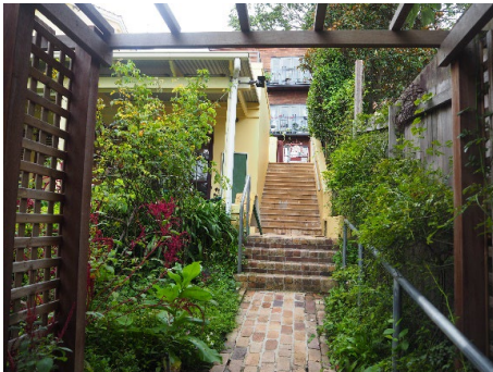
Figure 3. 20: The later addition entry steps running down the southern side of the tearooms building joining with the original brick path.
