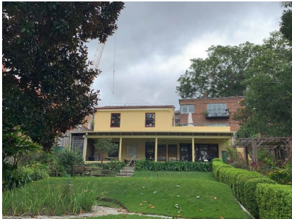
Figure 3. 110: Former garage and flatette
