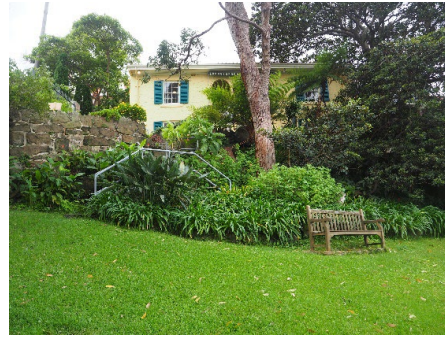
Figure 3. 67: View of west elevation as seen from the Lower Garden
