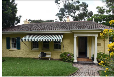
Figure 3. 60: Front (eastern) elevation, showing entry portico.
