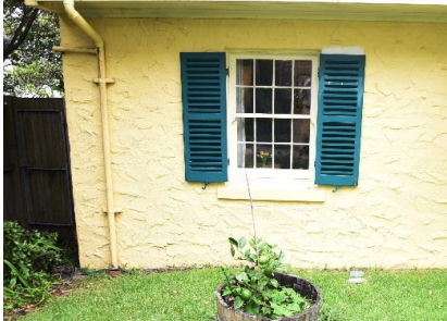
Figure 3. 62: Typical multipaned sash window with shutters
