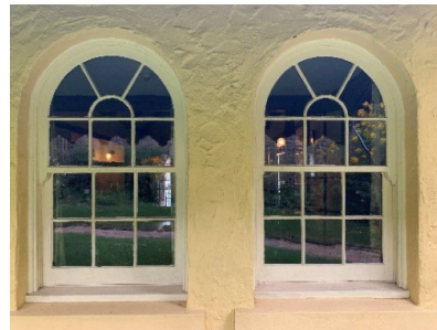
Figure 3. 63: Detail of multipaned round headed sash windows.
