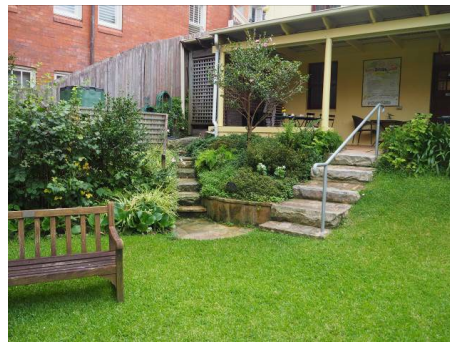
Figure 3. 23: North-western corner of the former Garage/Flatette with later addition stone steps.
