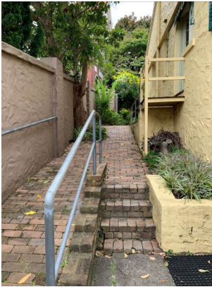
Figure 3. 29: Brick paved side path along northern side of the house.
