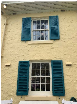
Figure 3. 68: Windows on west elevation with shutters
