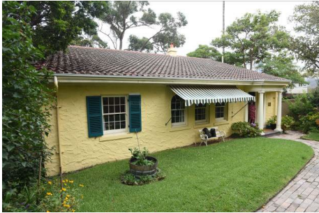
Figure 3. 59: Front (eastern) elevation
