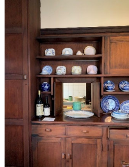
Figure 3. 89: Built in buffet with hatch to Kitchen
