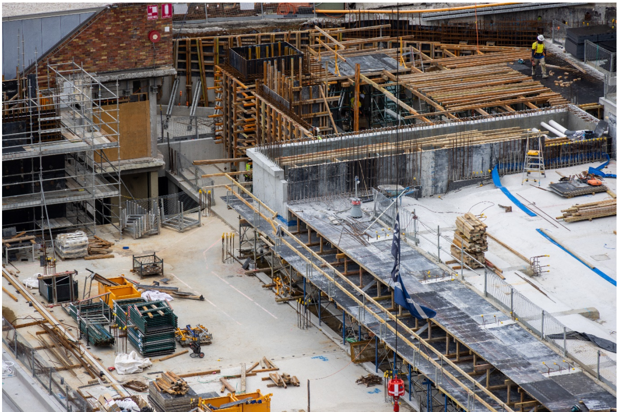
Plant room area under construction 20 December 2022
