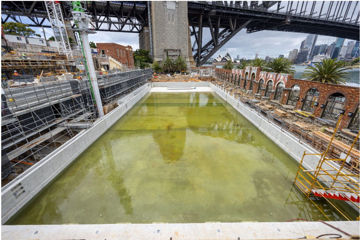
50m Pool has passed the leak test 20 December 2022
