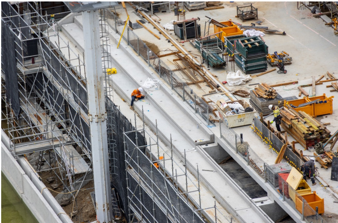
Lower Grandstand installation underway 20 December 2022
