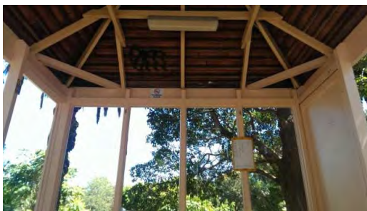
BS023: Interior Roof
