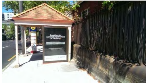
BS033: Southern elevation with electronic advertising board
