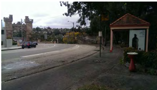
BS001: Looking north towards Bridge nominally 5m to the south of BS001
