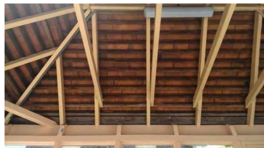
BS031: Interior roof
