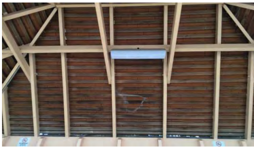
BS001: Interior of roof
