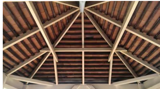
BS051: Internal Roof
