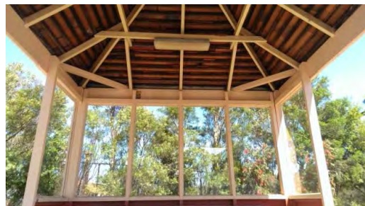
BS026: Interior Roof
