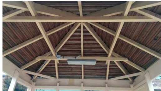
BS065: Internal Roof
