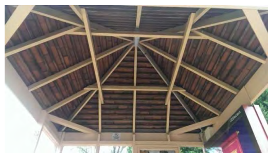
BS016: Internal roof
