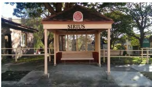
BS011: Front elevation, looking west
