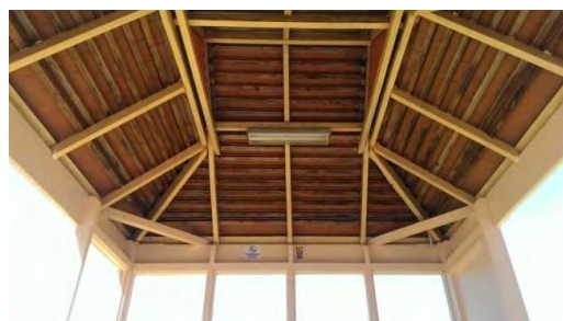
BS061: Internal roof
