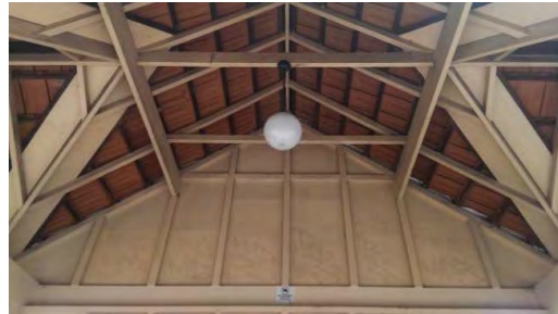
BS053: Interior roof
