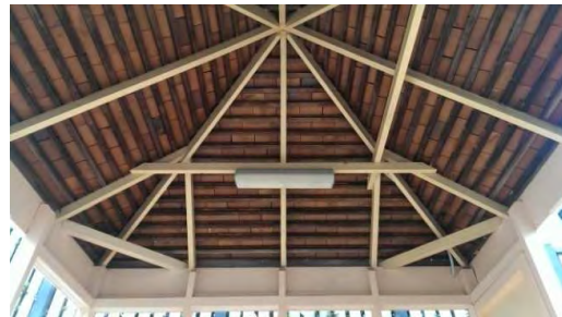
BS018: Internal roof
