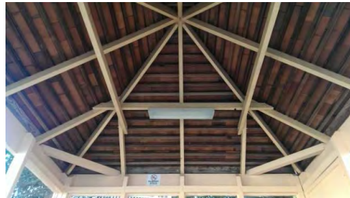
BS012: Internal Roof
