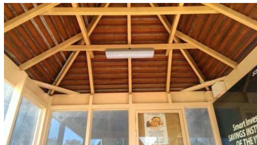
BS038: Interior roof
