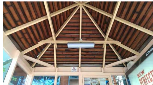
BS003: Internal Roof
