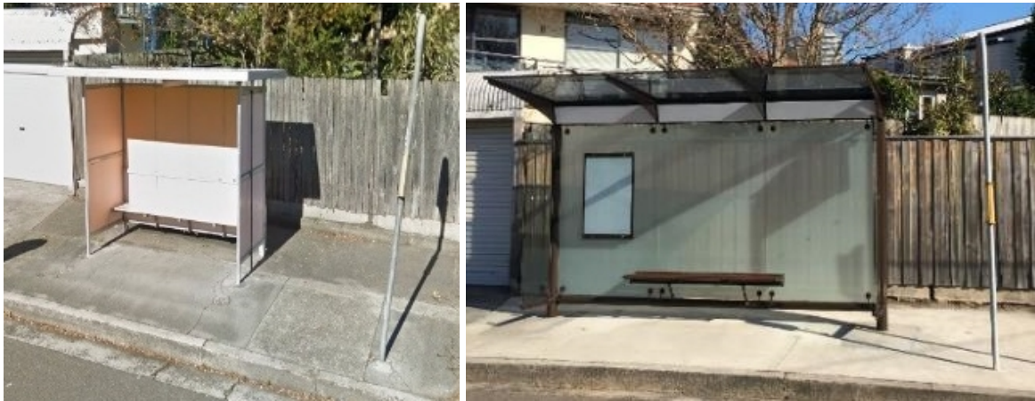
Before – After Benelong Road, Cremorne – also replaced in 2017
