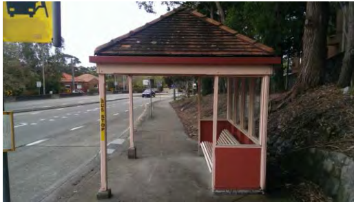
BS002: Looking north along Miller Street
