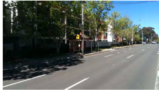
BS003: Street view looking south along Miller Street
