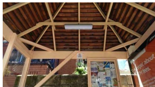
BS006: Internal roof
