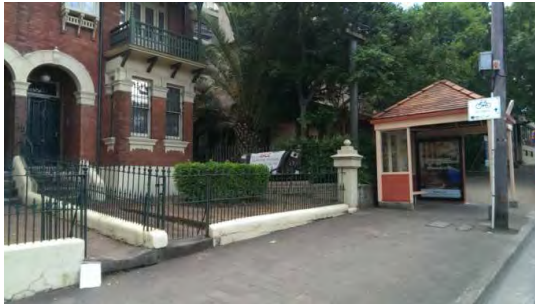
BS045: Adjacent buildings, looking north
