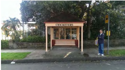
BS012: Front elevation, looking west
