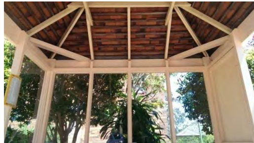
BS060: Interior back and roof
