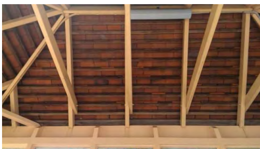
BS010: Internal Roof
