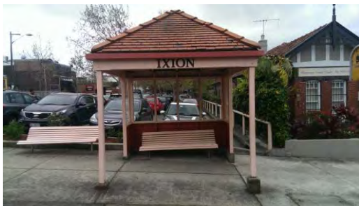
BS019: Front elevation, looking north
