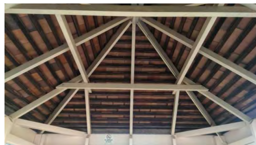
BS011: Internal Roof
