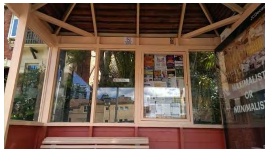
BS045: Internal roof
