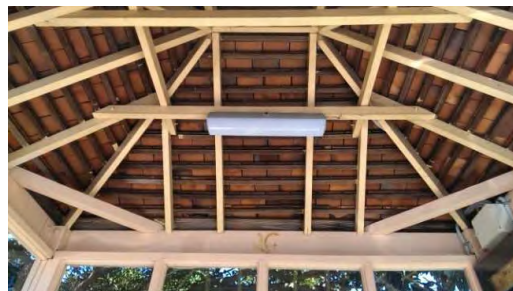
BS046: Interior roof
