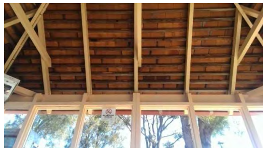
BS058: Interior roof
