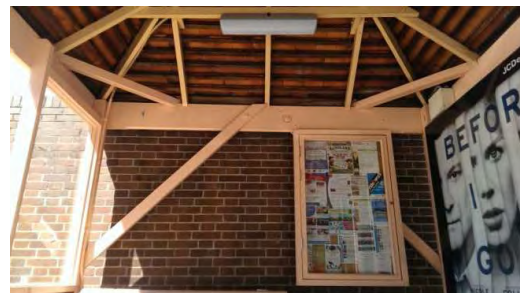
BS057: Roof and back wall
