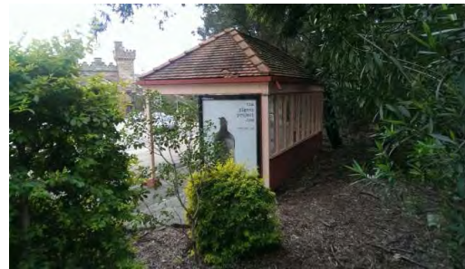
BS001: Southern/western elevations
