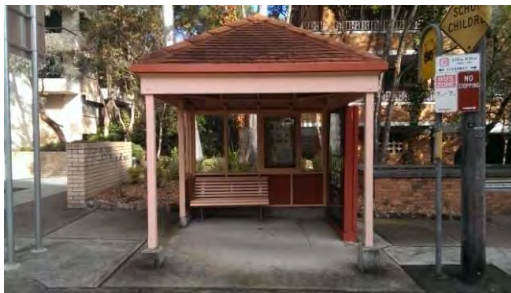
BS066: Front elevation looking south
