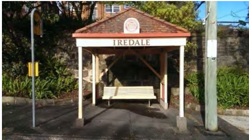
BS051: Front elevation, looking east
