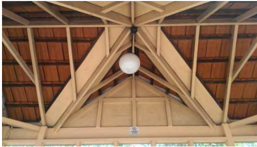
BS054: Interior roof and light
