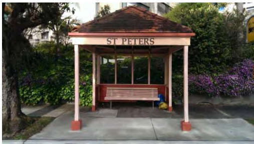
BS013: Front elevation, looking east
