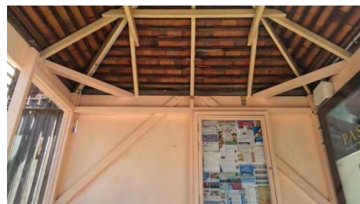
BS033: Interior roof
