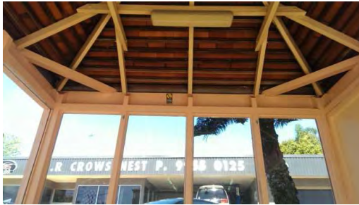
BS020: Interior roof
