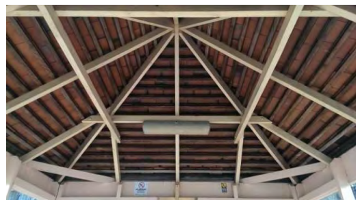
BS002: Internal Roof
