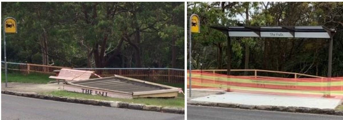
Before – After The “Falls” bus shelter in Cremorne was demolished by a truck in March 2022. The shelter was fully replaced with a Cox Type 4 Shelter as per Council’s Public Domain Style Manual in September 2022.
