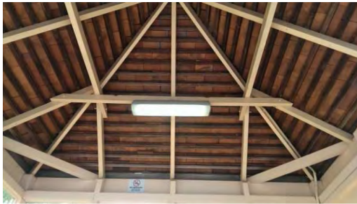
BS013: Internal roof
