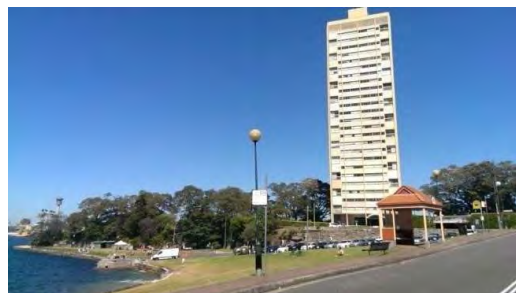
BS061: Street view, showing Blues Point Tower
