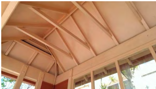
BS034: Interior roof
