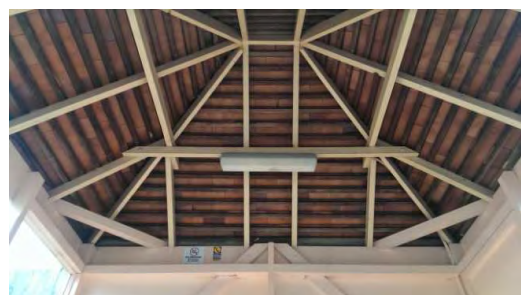
BS052: Internal roof
