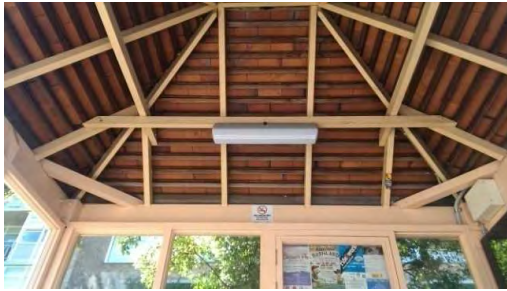
BS055: Interior roof
