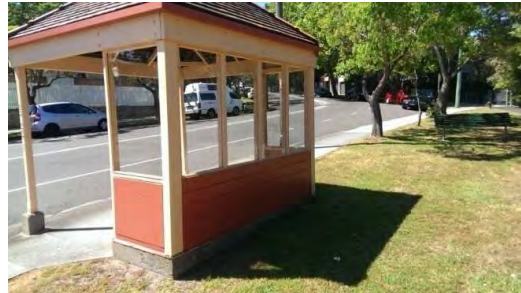
BS026: Southern and western elevations
