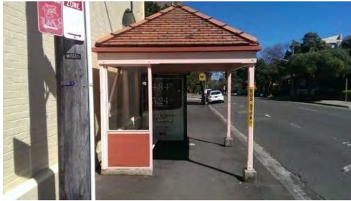
BS028: Northern elevation, looking south along Ben Boyd Road
