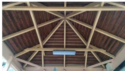
BS066: Internal roof
