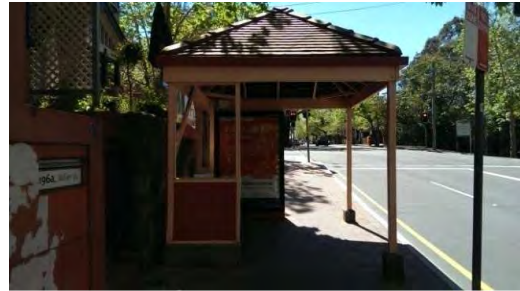
BS006: Looking north
