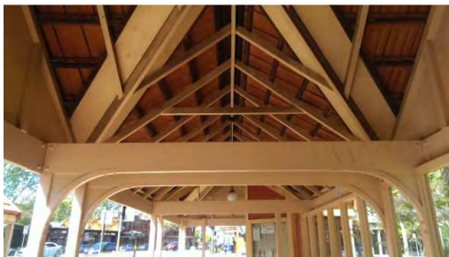
BS053: Interior roof
