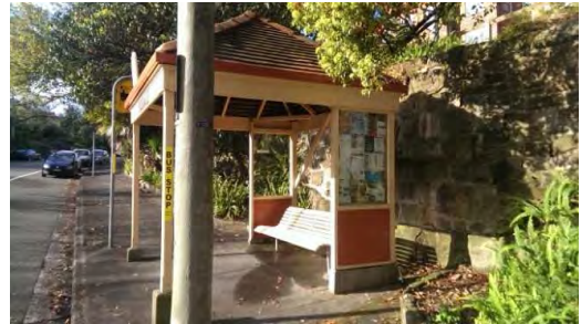
BS051: South elevation with community board
