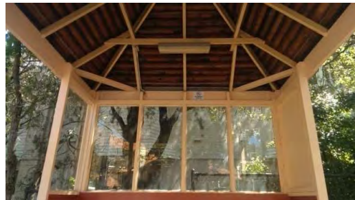
BS029: Interior roof
