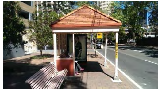
BS005: Northern elevation, with additional seat
