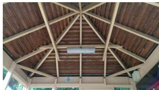
BS067: Internal roof
