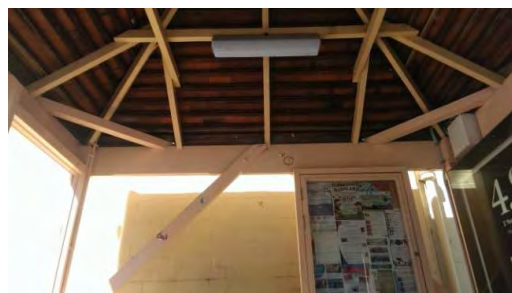
BS028: Interior roof
