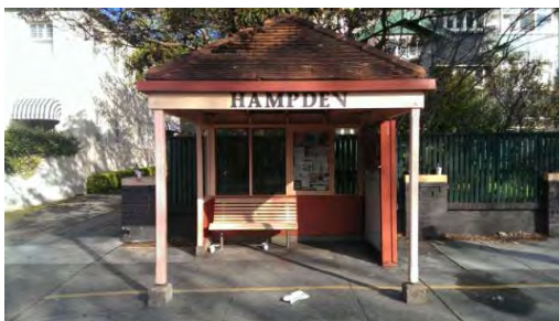
BS009: Front elevation, looking south
