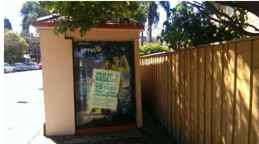
BS031: Southern elevation, showing electronic Advertising panel and closed in side wall
