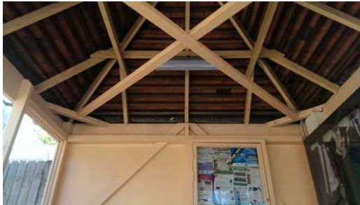
BS007: Internal roof
