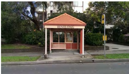
BS067: Front elevation looking south
