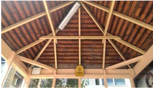
BS005: Internal ceiling
