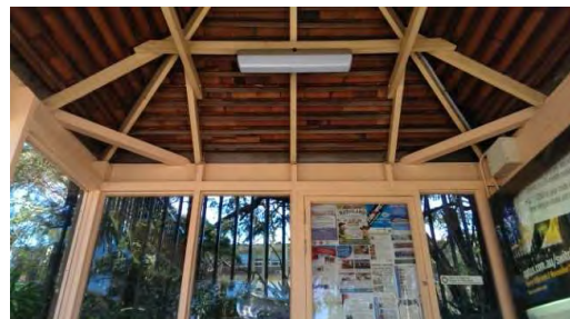
BS008: Internal roof
