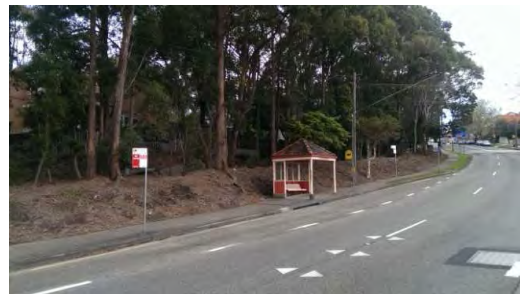
BS002: Street view, looking south
