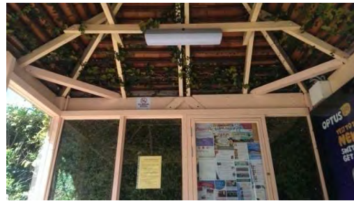
BS030: Interior roof
