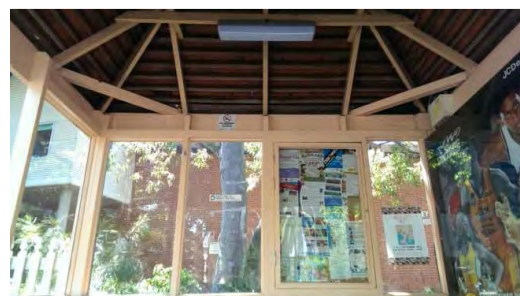
BS035: Interior back and roof
