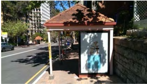
BS006: Northern elevation, showing advertising panel
