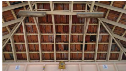
BS004: Internal ceiling
