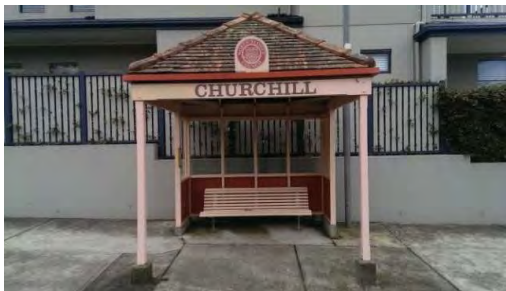
BS018: Front elevation, looking north
