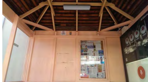
BS056: Interior Back and Roof
