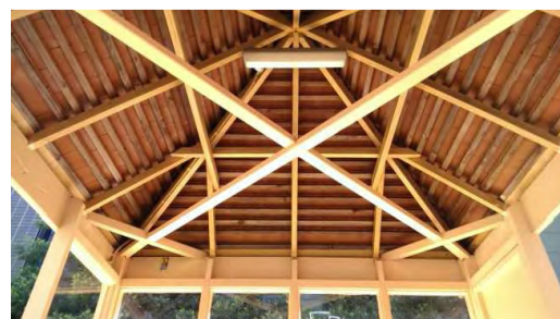
BS059: Interior roof
