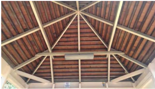
BS044: Interior roof
