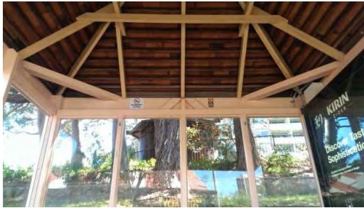
BS024: Interior roof
