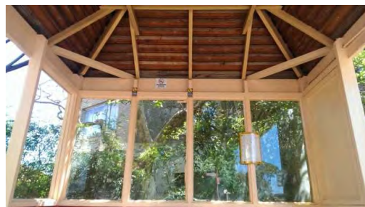
BS022: Interior roof
