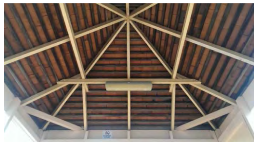
BS019: Internal roof
