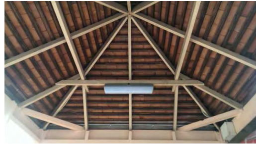
BS009: Internal Roof
