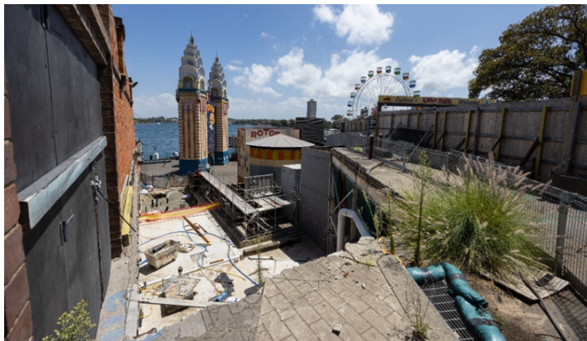
Western Stairs Slab 6 February 2023
