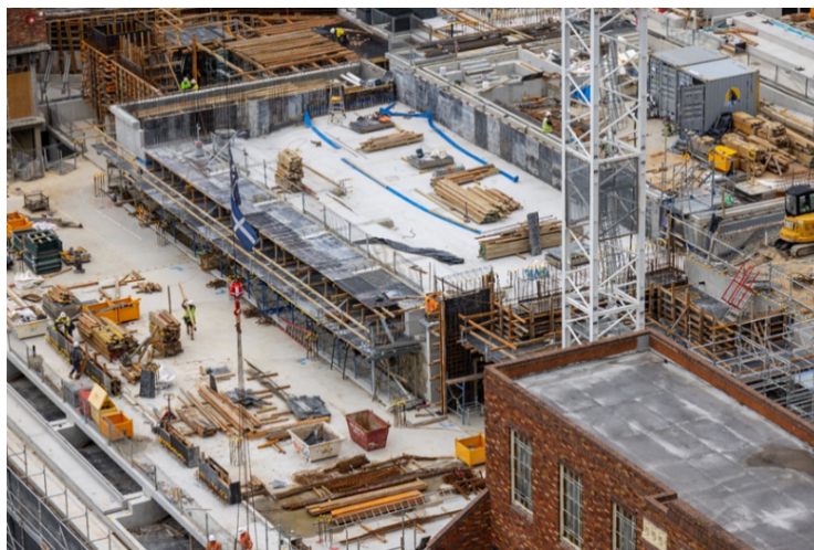
25m Pool base and walls under construction 20 December 2022
