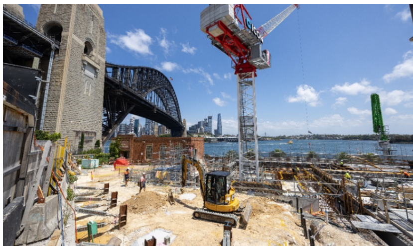
NE corner Level 3 6 February 2023
