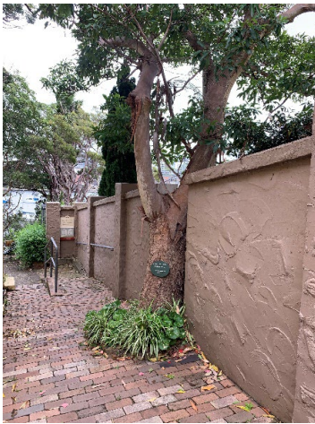
Figure 3. 47: Roughcast rendered masonry wall adjacent to the Main House
