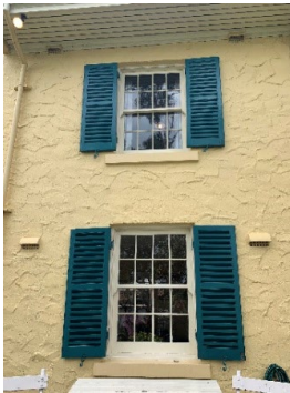
Figure 3. 68: Windows on west elevation with shutters
