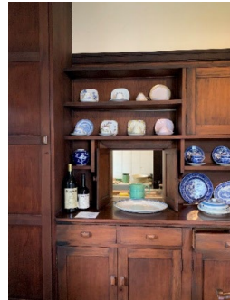
Figure 3. 89: Built in buffet with hatch to Kitchen
