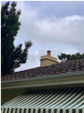
Figure 3. 64: Chimney and roof pan tiles
