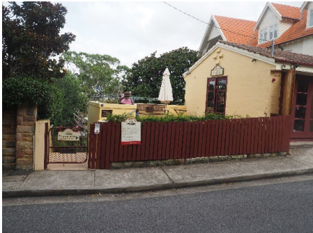
Figure 3. 45: Front fence and gate
