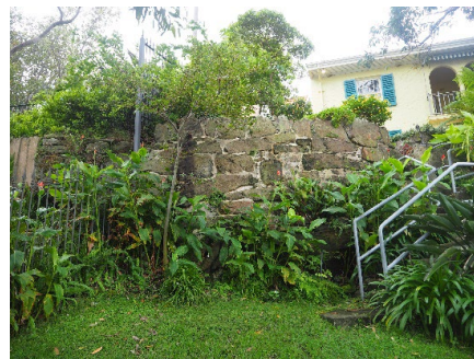
Figure 3. 34: Sandstone retaining along northern side of the terrace area above. Note metal handrails for central steps.
