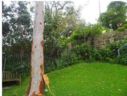
Figure 3. 48: Later addition metal palisade fencing on northern boundary
