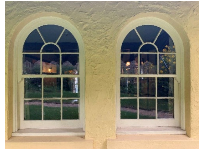
Figure 3. 63: Detail of multipaned round headed sash windows.
