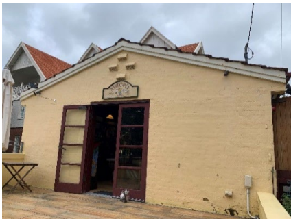
Figure 3. 112: Southern entry into former garage from viewing platform/terrace.
