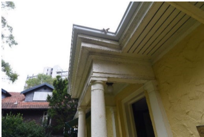
Figure 3. 61: Soffit and portico
