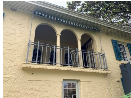
Figure 3. 70: Loggia with balustrade
