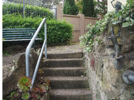
Figure 3. 36: 3. 37: Concrete and stone steps with metal handrails connecting House Terrace to Lower Garden with rockeries.
