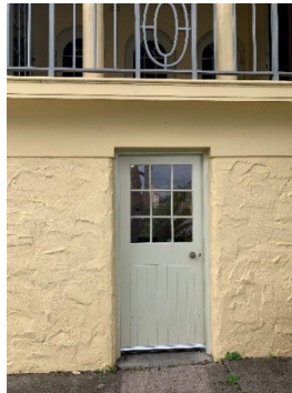
Figure 3. 69: Door into the lower level on west elevation
