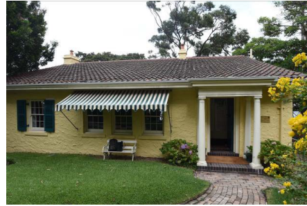
Figure 3. 60: Front (eastern) elevation, showing entry portico.
