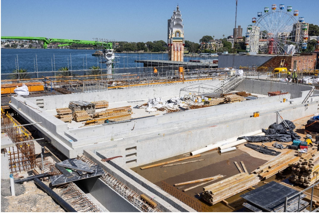
25m Pool base and walls complete 7 March 2023
