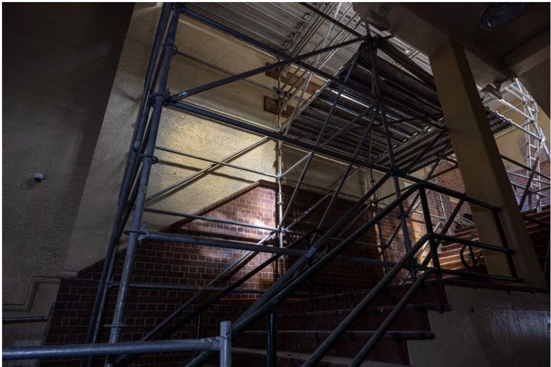
Inside the Eastern Stair Tower 7 March 2023
