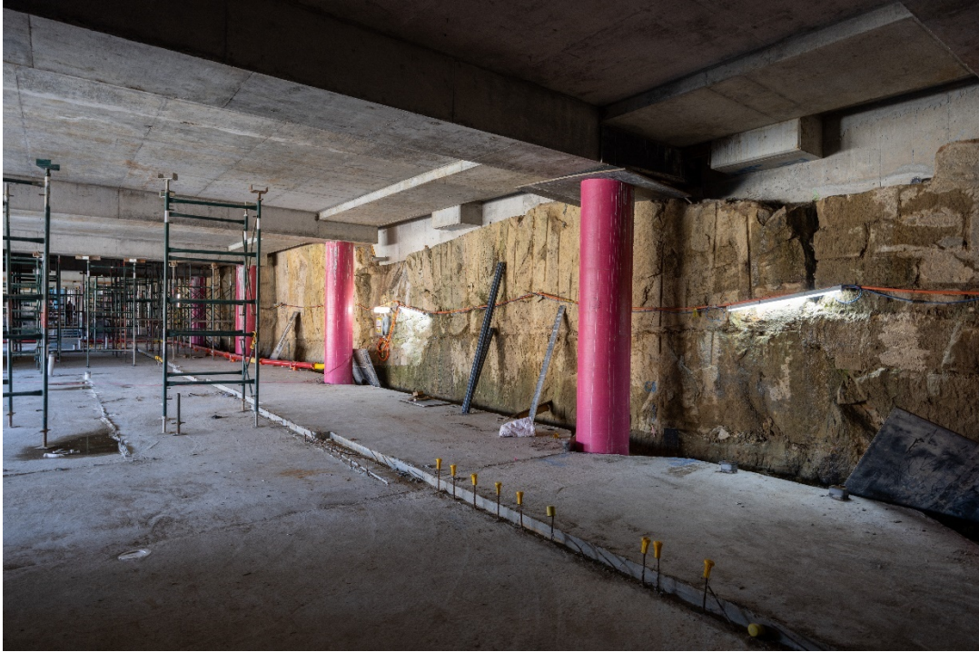
Level 1 amenities area stripped 7 March 2023
