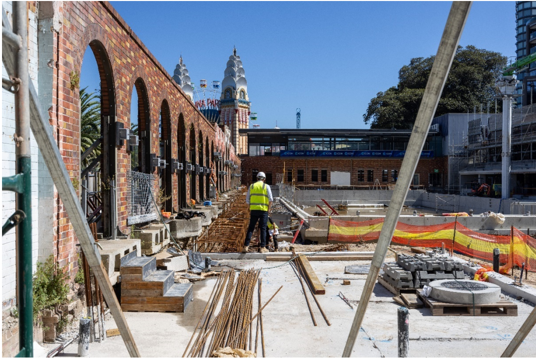
Ripples kitchen slab poured 7 March 2023
