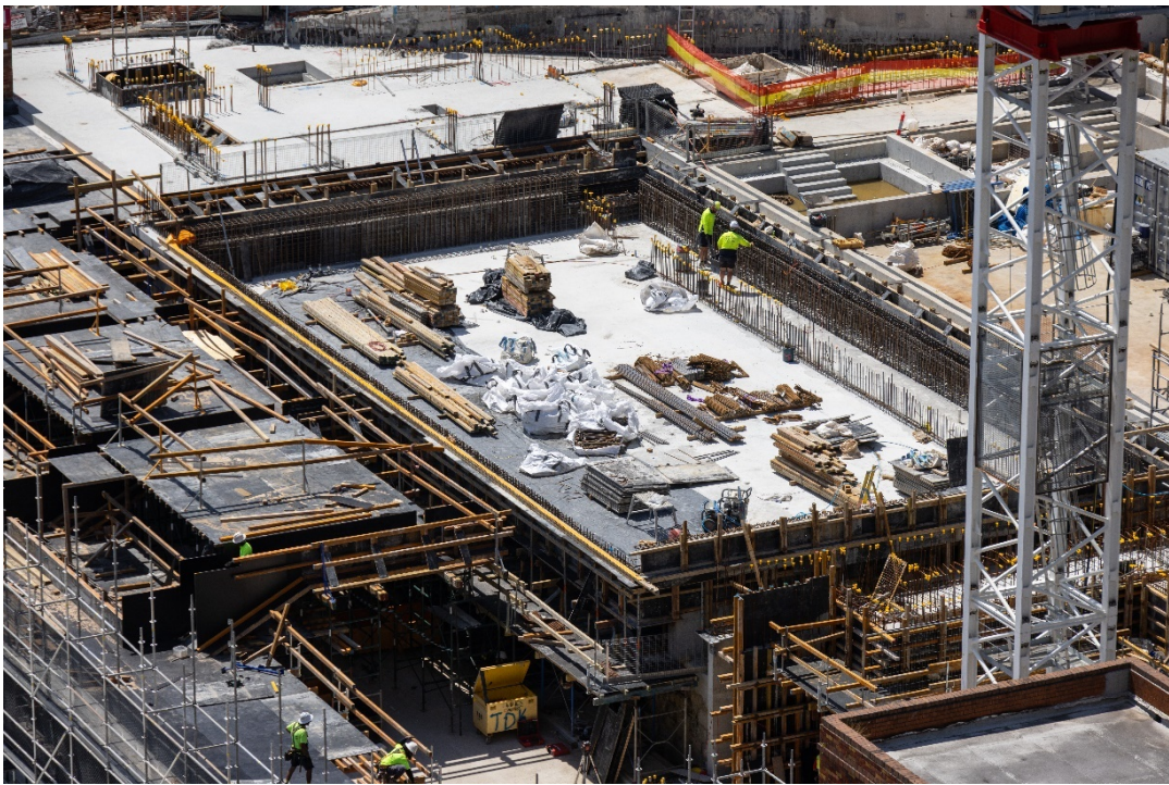
25m Pool base and walls under construction 6 February 2023
